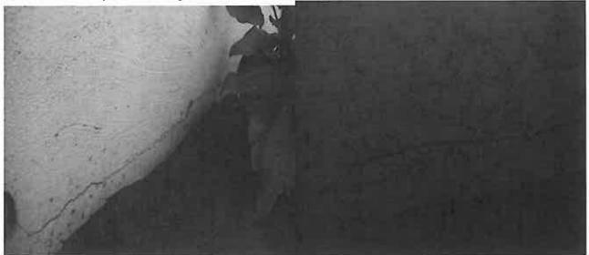
• Improve: Peeling paint was noted on the exterior of the home in various areas. This can lead to moisture related issues. Repairs are recommended.
