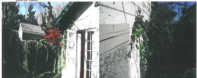
Repairs: Cracking on the exterior walls near the top of the foundation are signs of possible settlement. Further
