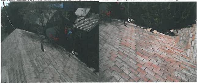
• Repair: Damage of the asphalt roof covering was noted. This type of damage is likely to cause roof leakage at this location and requires repair. Further evaluation and repair by a qualified roofing contractor is recommended.
