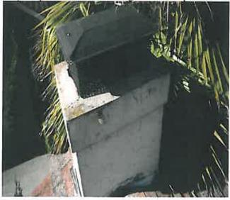
• Improve: The mortar cap at the top of the masonry chimney has several minor cracks. While this damage is considered to be minor, and commonly found, the cracks should be sealed to prevent moisture intrusion into the brick and mortar. Repairs by a masonry contractor or other qualified trades person is recommended.
