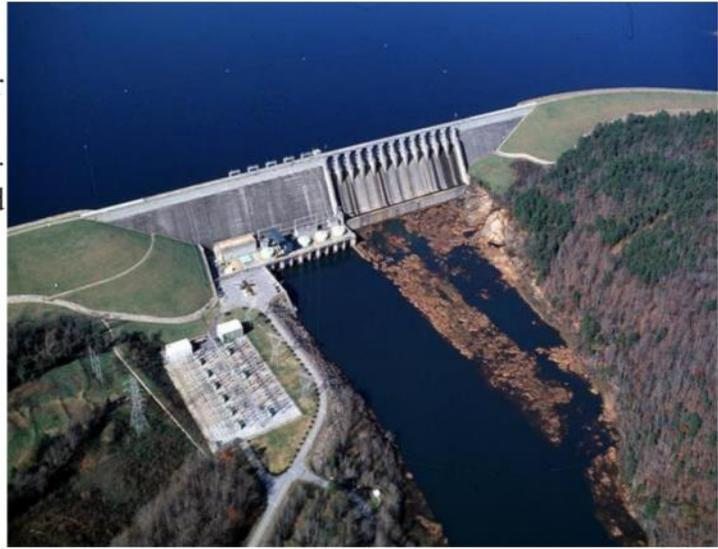
The power plant originally consisted of four generators, with provisions made for a 5th generator based on the foresight that additional power demands would be likely. The 5th generator was installed in 1983. The Hartwell Project power plant has the distinction of being the only hydroelectric plant to be totally designed and constructed by the Corps, with the generators located outdoors.
