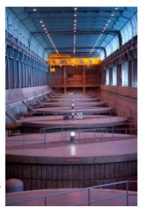
However, in addition to the four conventional turbines already on line for power production at the Russell Dam, the power plant has four reversible pump-storage turbines, known as pump back units. The four pump back units at Russell Dam are different than regular generators in that at night, when electrical power demands are low, they can operate in reverse direction to pump water from below the dam back upstream into Russell Lake.
