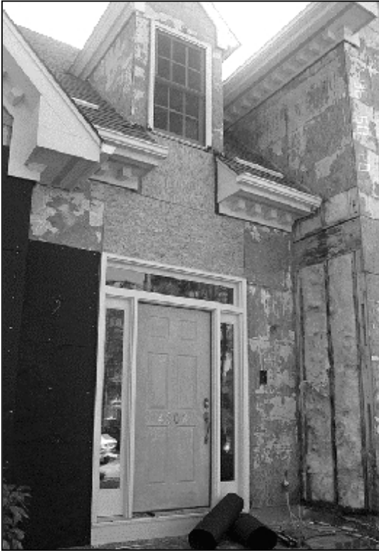
Decay discovered in a wall and floor band below a rake (kick out) flashing area.
