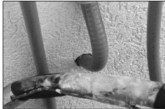
Electrical conduit penetrates without sealant.
