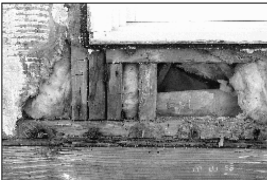
Extent of decay in studs can be assessed with an awl.
