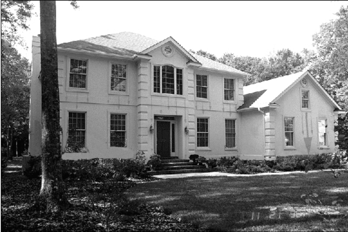
Figure 6 Upper Level Windows
