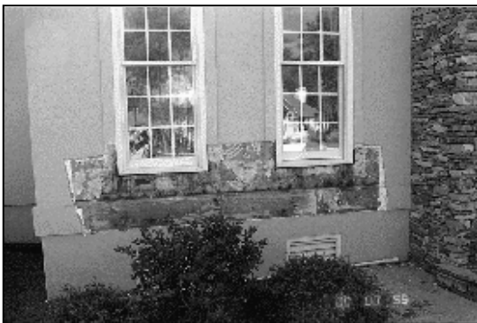
Small opening in window construction allowed a large quantity of water to enter a wall resulting in rot.
