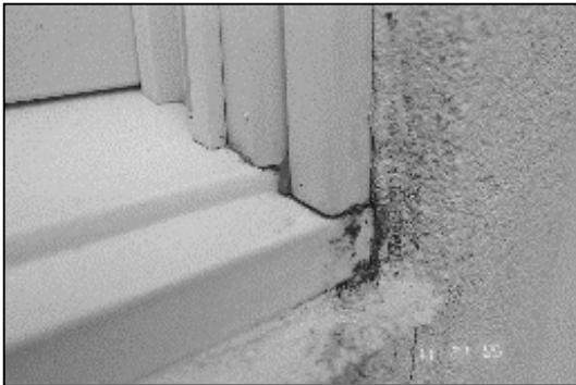
Window frame leaks at the corner of sill and jamb connections are "typical" of some windows.
