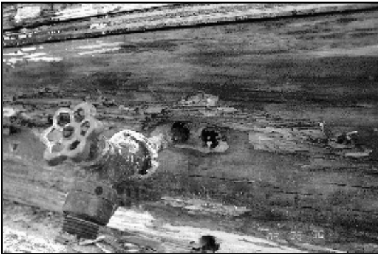
Decay of a 2x10 band from a hose bib penetration.
