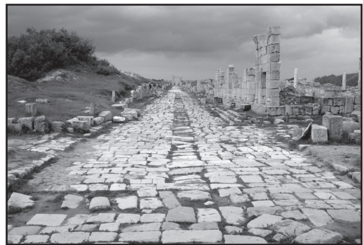
Road built by Rome in the ancient city of Leptis Magna, Libya. Dirk.heldmaier. Used under Creative Commons Attribution-Share Alike 3.0 Unported license.
