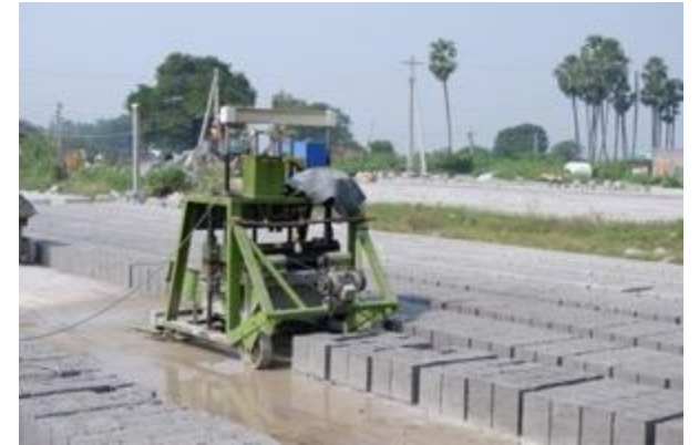
Fly Ash Brick Manufacturing Unit
