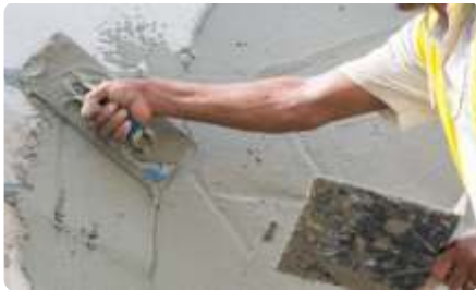
Figure 221: Plastering in progress Source: N.Srinivasa, 2019
