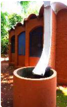
Figure 180.1 The rainwater being collected into a small tank in Vikas Community
