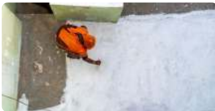
Figure 227: Waterproofing paint for the roof Source: BBC
