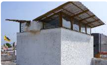
Figure 205: Slanted sheds featuring water collection in the beam
