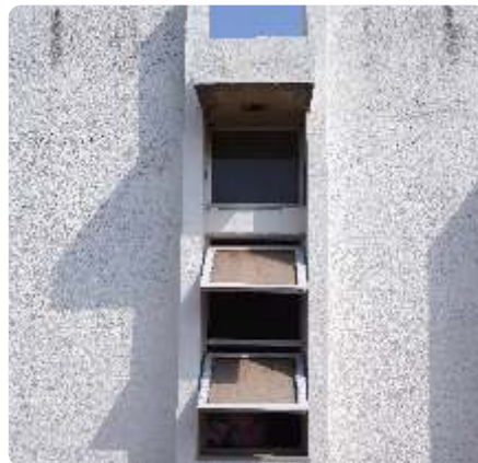
Figure 210: Window overhang with 1.5' depth
