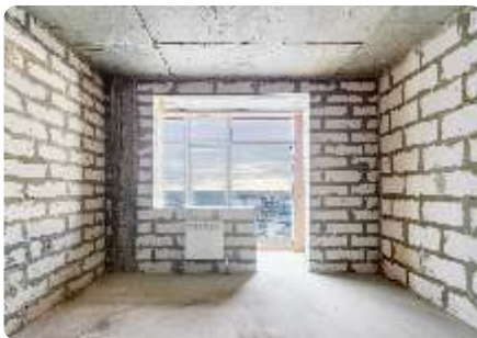
Figure 149: Wall construction with Autoclaved Aerated Concrete Source: Adobe Stock Image
