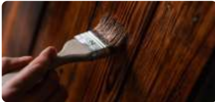
Figure 226: Priming the wood surface Source: Freepik
