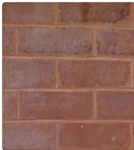
Figure 144: Wall constructed with CSEB Blocks Source: Adobe Stock Image
