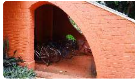
Figure 177: CSEB Blocks as Walling Material
