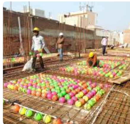
Figure 114: Bubble Roof Deck Source: Ashok B. Lall Architects
