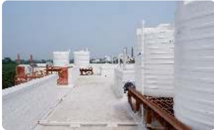
Figure 254: White Paint on the Roof
