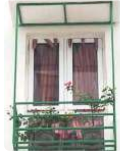
Figure 167: Cement Board overhang with MS Frame Source: Building Envelope solutions sets (V.10) for eco-niwas samhita 2018
