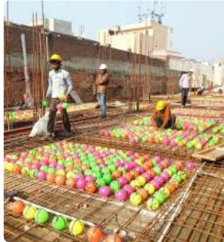
Figure 130: Construction of a bubble deck Source: Butterflies Resilience Centre, Ashok B Lal
