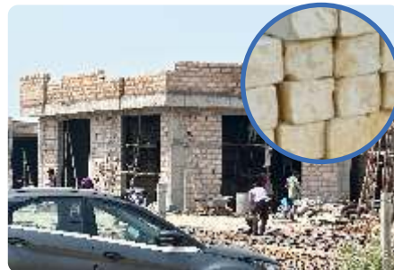
Figure 202: Construction with Bela Stone in Progress
