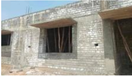
Fly-ash used as walling material in Andhra Pradesh
