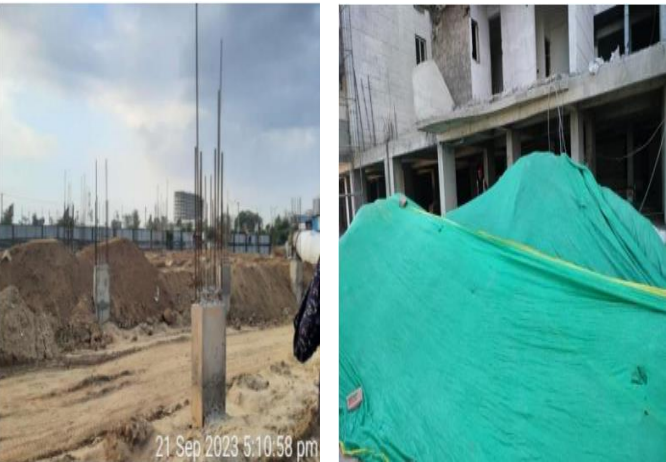
Before (No covering over fine construction materials) After (Covered stock-piling of excavated topsoil)
