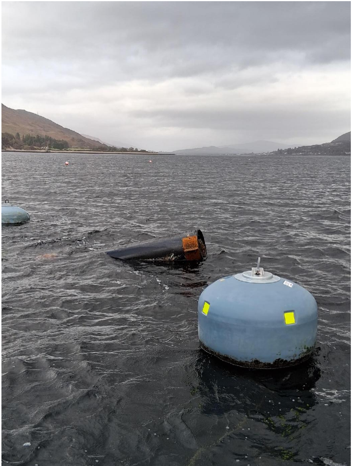
Photo 4: Most eastern end of the tidal barrier floatation tube, partially sunken with a metal fixing (which was used to secure the floatation tube to the cage group using chains).
