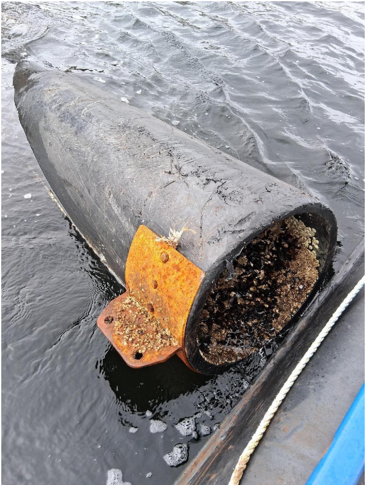
Photo 5: Close up of the eastern end of the floatation tube with metal fixing.
