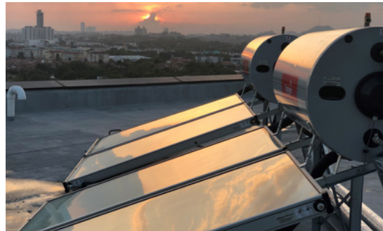
Panama | Apartment Complex
