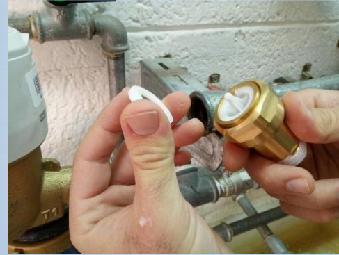
Placing the seal on top of the LFC
