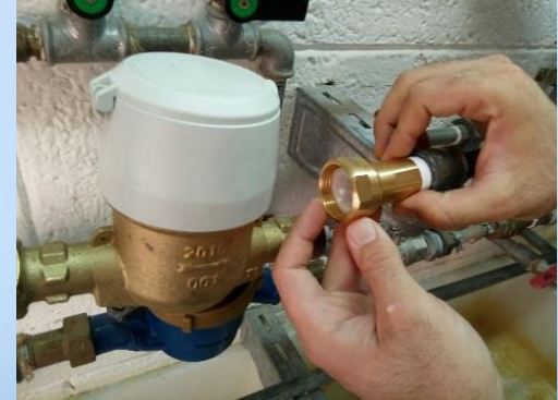
Screwing the LFC into the water meter
