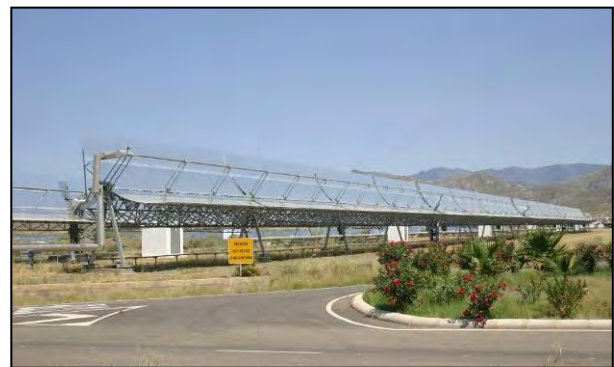
(b) Direct Steam Generation (DISS) test loop – 300m of ET II trough, 5.78m width, 12m long modules
