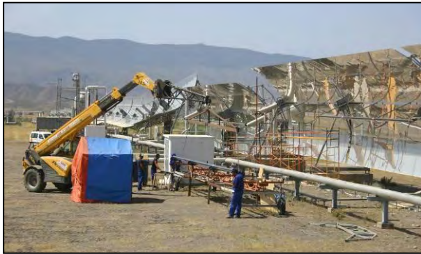
(c) Changing receivers on the DISS loop, note the use of a small off road capable telescopic crane.
