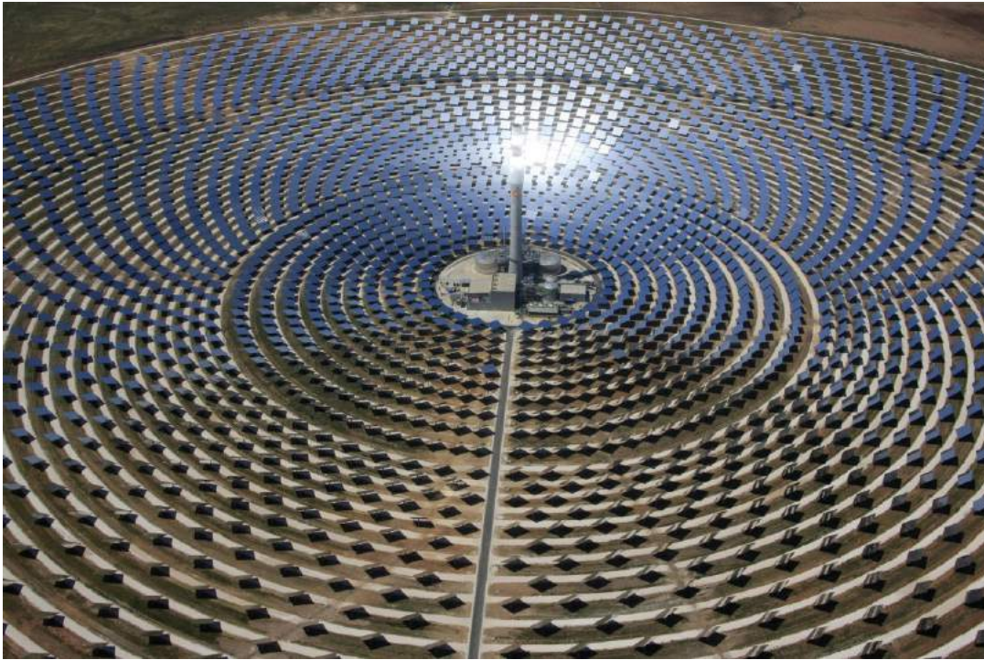
Figure 44. Aerial view of the Gemasolar Heliostat power tower plant in Spain, thermal capacity 400\text{MW}_{th} (courtesy of Torresol Energy).
