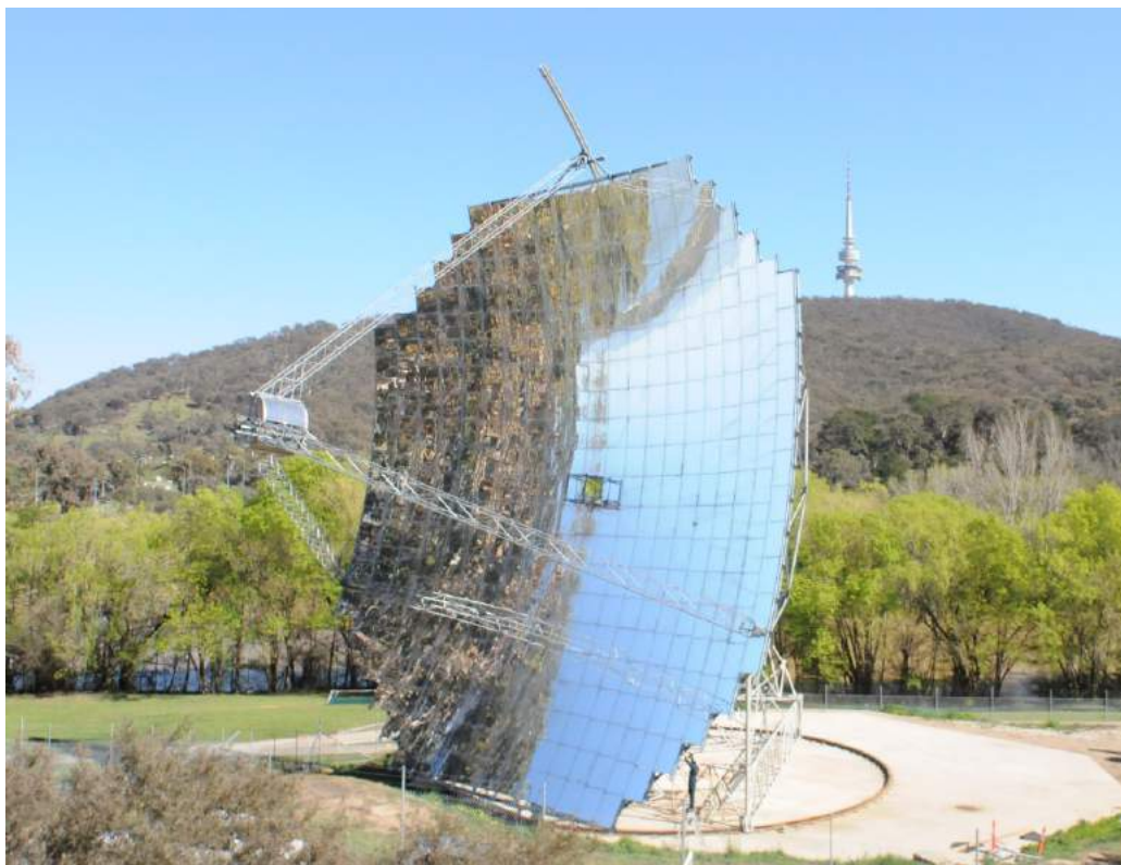
Figure 45. Australian National University's prototype 500m 2 paraboloidal dish concentrator (picture K Lovegrove)..
