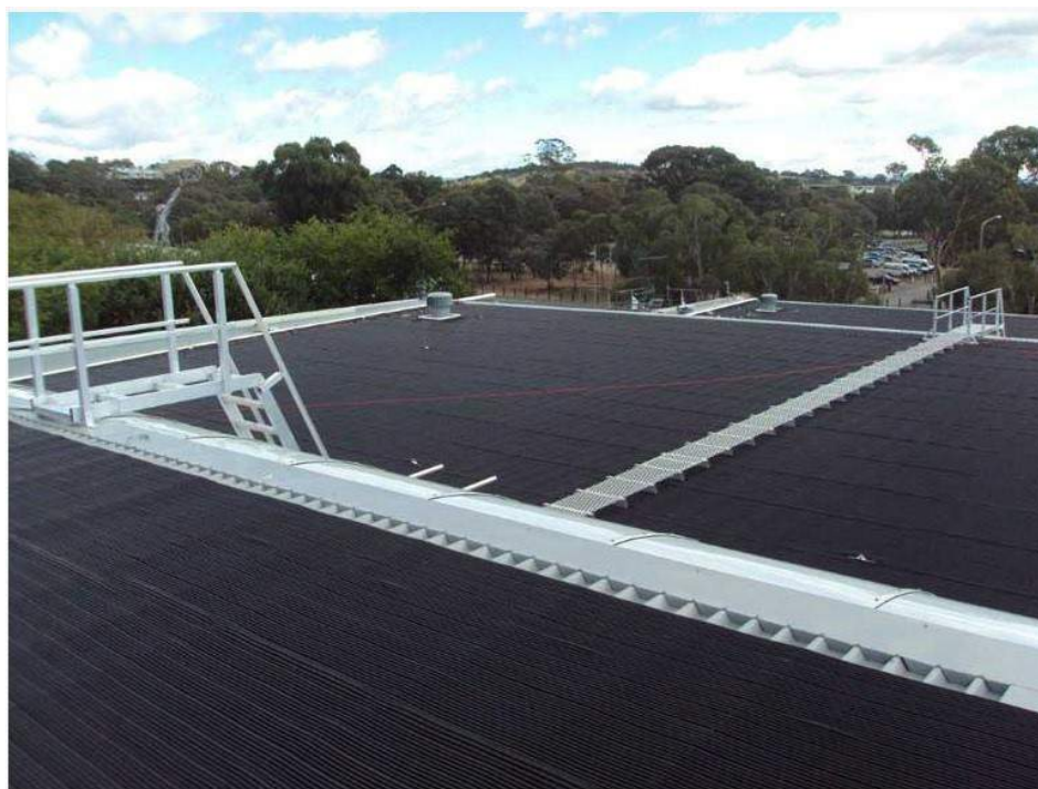
Figure 30. Unglazed Collector for an indoor pool at the Australian Institute of Sport, Canberra 17
