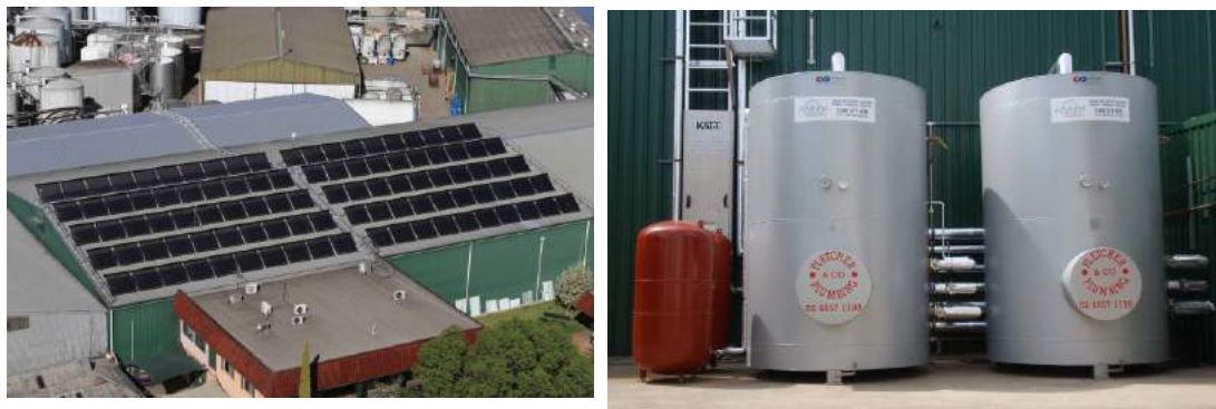
Figure 59. Evacuated tube collectors and storage tanks, photos Apricus
