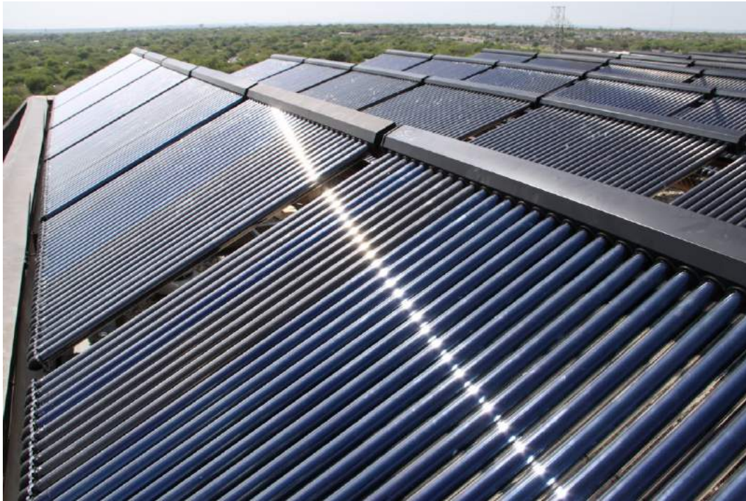
Figure 34. Evacuated tube collector array 21
