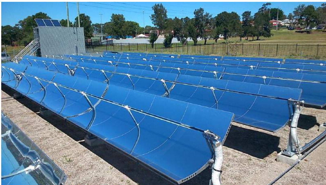
Figure 41. Small aperture parabolic trough collector (picture from NEP)
