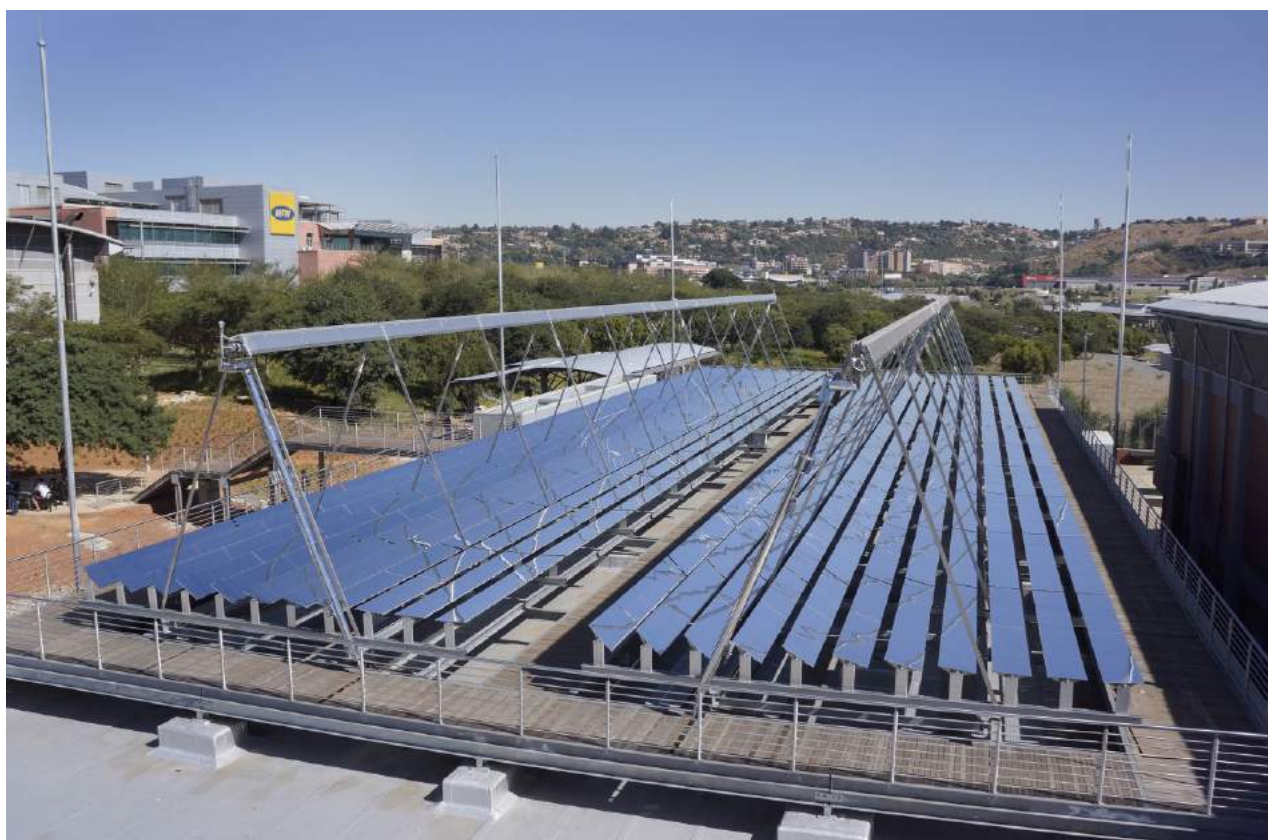
Figure 42. Linear Fresnel Collector (courtesy of Industrial Solar)
