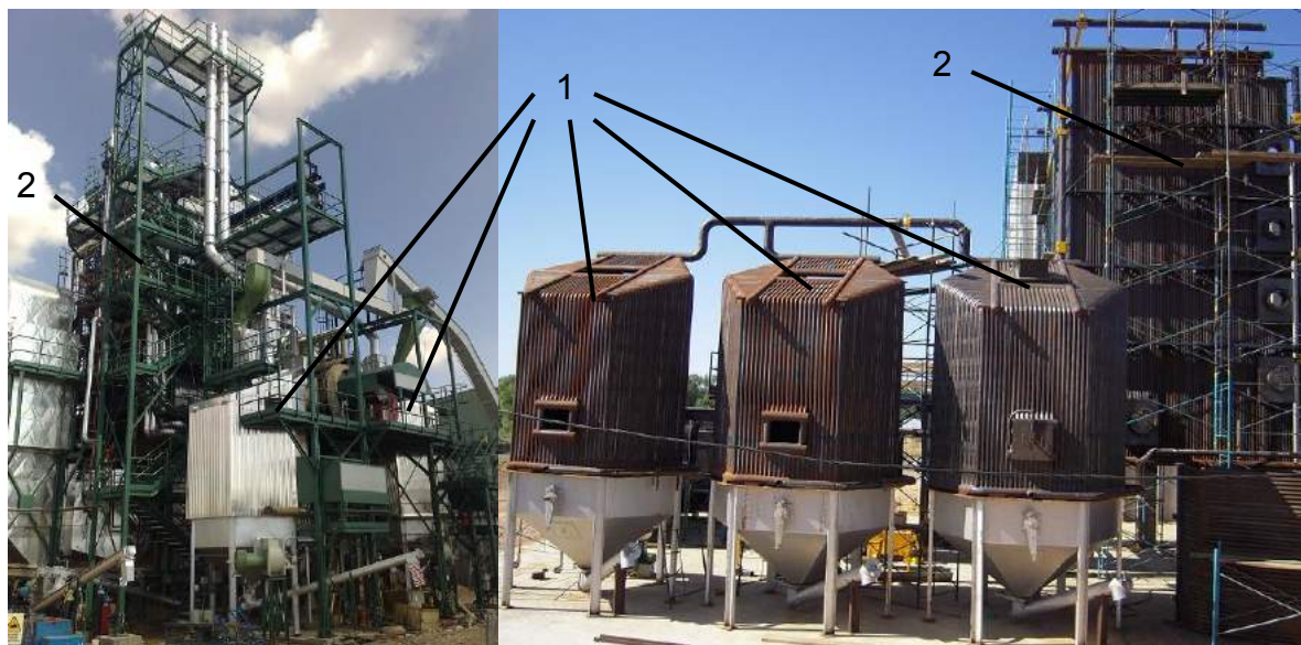
Figure 21: Boiler systems with two gasifiers (left) and three gasifiers (right) 12 . Gasifiers; 1, boilers; 2.
