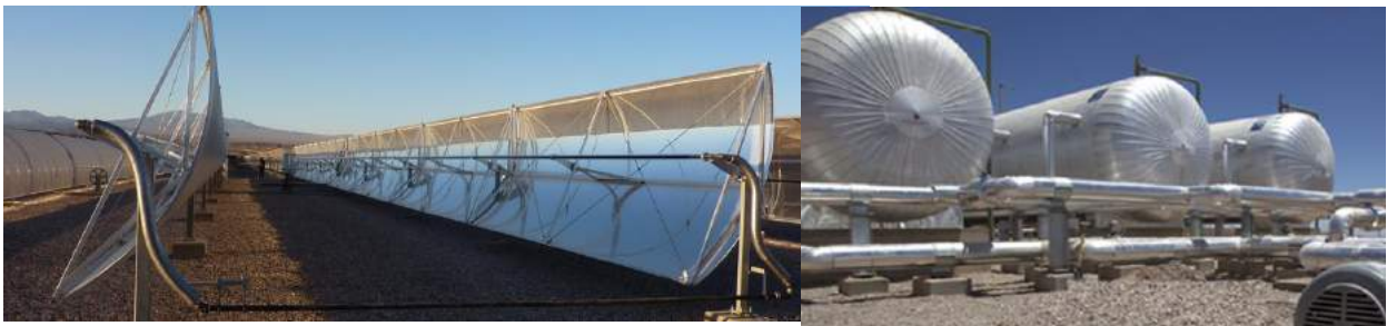
Figure 61. Parabolic trough collectors and thermal storage tanks at Minera El Tesoro, photos Abengoa Solar
