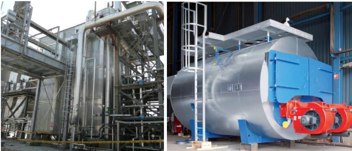
Figure 16: Natural gas fired water tube (left) and fire tube boiler systems (right) courtesy of Weismann Group
