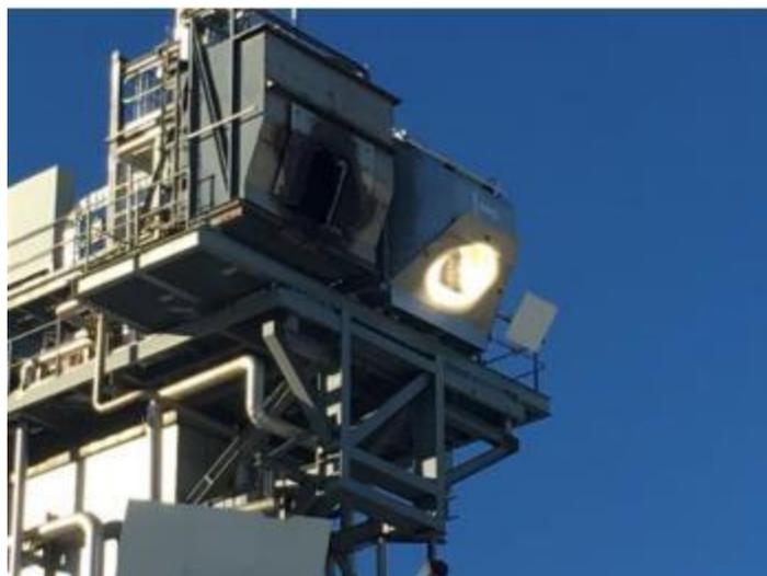
*On-sun operation of sCO<sub>2</sub> solar receiver at CSIRO's tower facility, Newcastle, NSW (image: CSIRO).*
