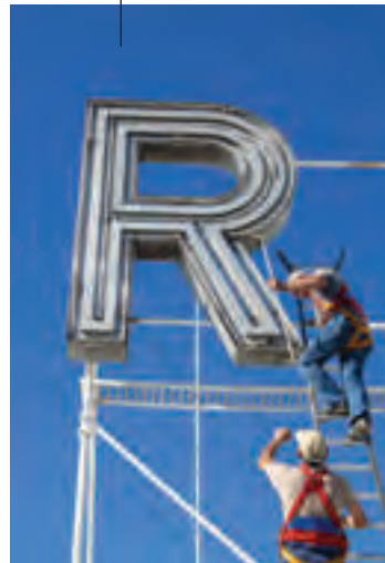
Taking down the letters of the Ritz Hotel was only possible with the help of lighting and signage company Neolux. Several teams were needed for the logistics of rescuing the letters. Each letter was 2.5 metres tall, weighed 80 kg and had to be lowered from a 10-storey building of one of the city’s most emblematic hotels.
