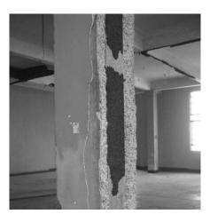
Figure 2 – Significant corrosion in concrete encased steel internal column in Central Point building
