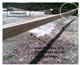
Figure 4 -Contraction joint making device developed by University of Moratuwa
