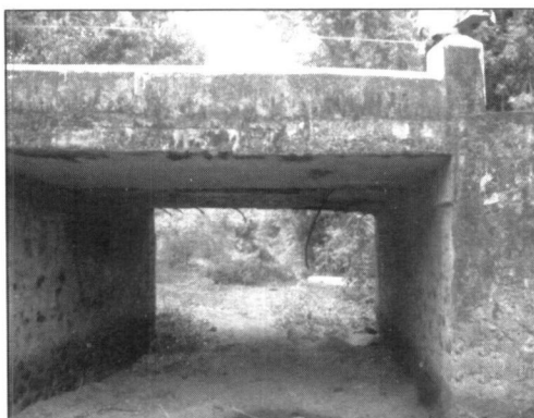
Figure 8: A side view of the case study bridge
