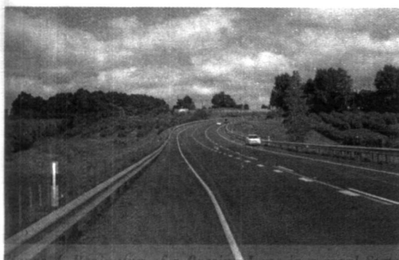
Figure 4. Beginning of a Passing Lane in a rural State Highway in New Zealand
