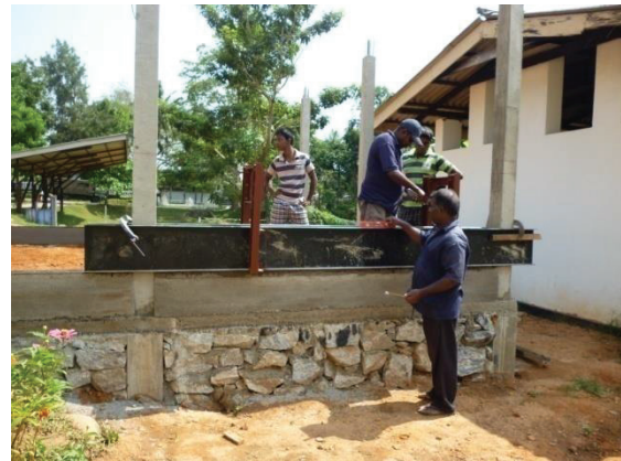
Figure 4 - NERDC Conventional Slip Form Wall Construction Technology
