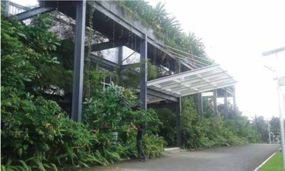
Figure 4: A Carbon Neutral Apparel Factory
