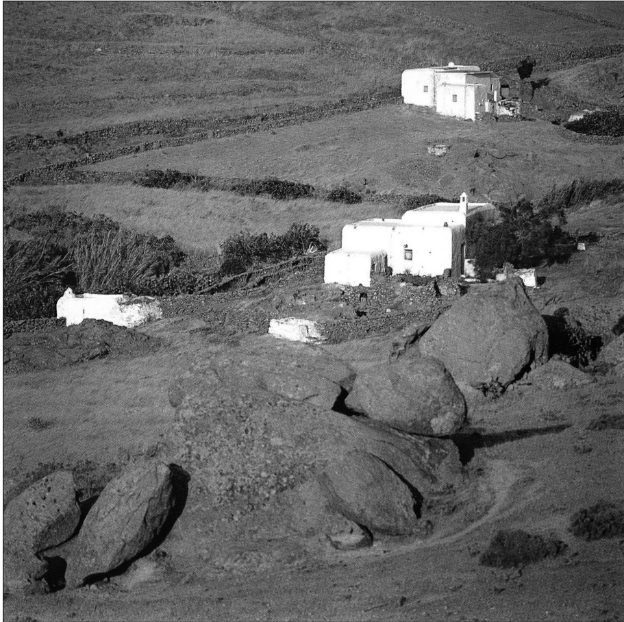
Figure 4: The 'choria' (permanent farmhouses) representing the 'true' vernacular architecture of Mykonos and its people were among those idealised by Aris Konstantinidis. [Courtesy of Philippides D (ed.). Greek Traditional Architecture , Vol. II. Athens, 1983: 51].
