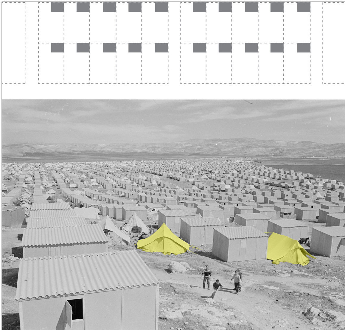
Figure 5: Photograph/diagram of the 1950s camp layout in Baqa'a showing UNRWA's grid layout of 96–100 m 2 plots, and with each plot having a 12 m 2 prefabricated room for the family to live in [Courtesy of UNRWA-ICIP Archives + drawing by the author].
