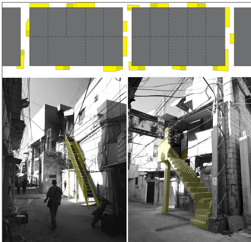
Figure 9: Photograph/diagram of the 1980s–90s camp layout in Baqa'a which, with the horizontal plane now saturated, the refugees adopted architectural elements to allow for vertical expansion. Light metal stairs (left) gradually morphed into solid, concrete stairs (right) [Courtesy of UNRWA-ICIP Archives + drawing by the author].
