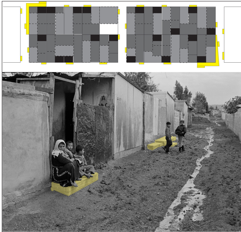
Figure 8: Photograph/diagram of the 1970s camp layout in Baqa'a showing that most refugee plots were now filled with concrete rooms, and thus concrete had started to overflow outside the plots in the form of Attabat ('doorsteps') which kept out muddy water and served as outdoor social spaces [Courtesy of UNRWA-ICIP Archives + drawing by the author].
