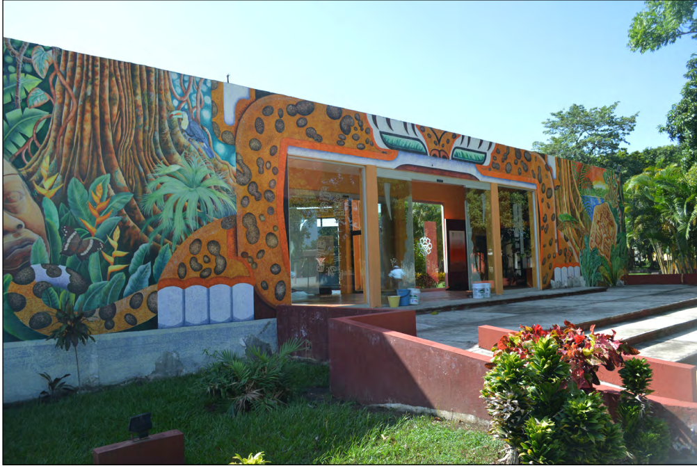
Figure 5 Façade of the Museo de Sitio de Tres Zapotes after being refurbished in 2007. Photograph by the author.
