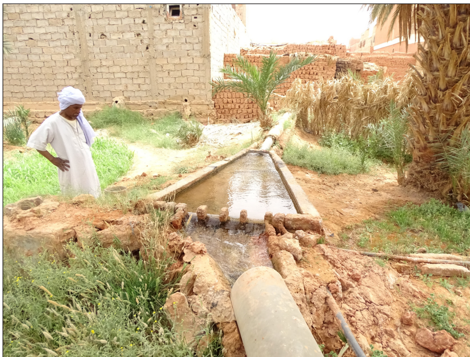
Picture 3 Replacing traditional channels by modern pipes while keeping the use of the water sharing basin ( kesria ) to ensure the visibility of water distribution for all. On the picture, the channel upstream of the kesria (top of the picture) has been replaced by a concrete pipe carrying all of the discharge of the foggara. In the kesria , part of the foggara discharge is diverted to smaller pipes that go left and right on the picture. What is remaining is the combined discharge of several water owners that will be transported in the big concrete pipe further downstream, where there is another kesria to sub-divide between these owners. (April 2017).
