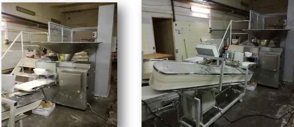
Figure 1: Bakery operation – Production hall - technological equipment - Hopper, Sliding belt.
