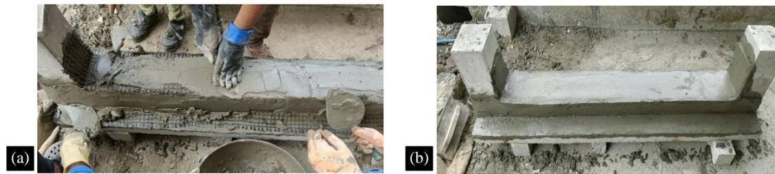
**Figure 7.** (a) Application of second layer of mortar and (b) Beam wrapped with FRCM.
