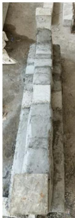
**Figure 9.** Application of FRCM in two layers.
