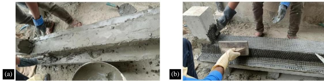
**Figure 6.** (a) Application of first layer of mortar and (b) Placing of fibre mesh.
