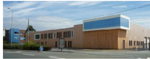
Fig. 1. The C.E.C.P/CEREMA building
