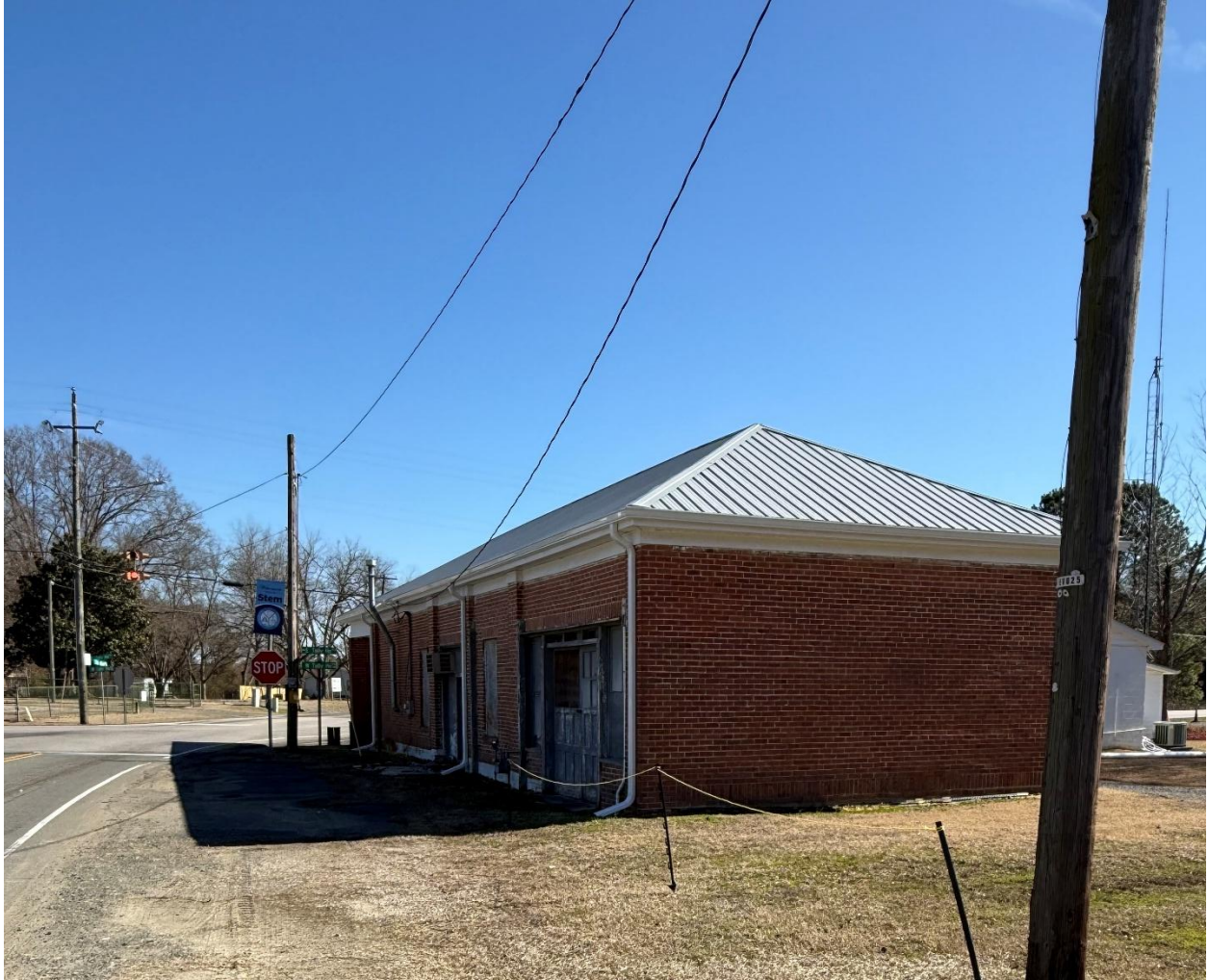
Rear of Mercantile Building
