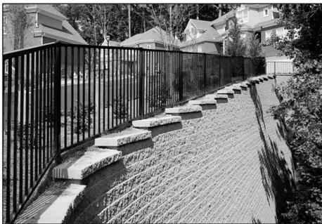
Often fences, stair rails, guide rails, or concrete traffic barriers are needed behind a VERSA-LOK wall. With proper design and installation, a variety of structural and aesthetic features can be placed at the top of a VERSA-LOK wall.
