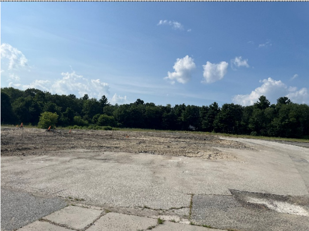
#5 Building demo and debris removal complete
