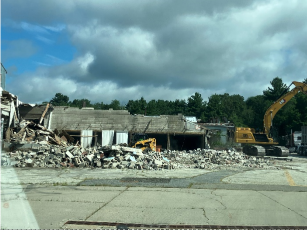
#1 Building demo progress
