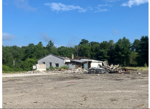
#2 Building demo progress
