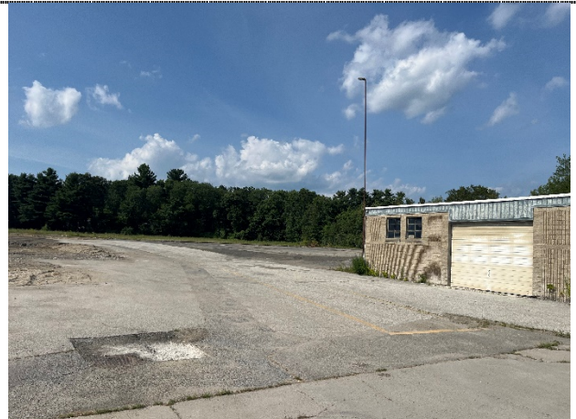
#6 Building demo and debris removal complete
