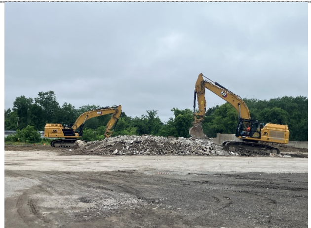
#4 Building debris removal progress
