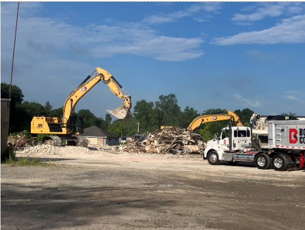
#3 Building debris removal progress
