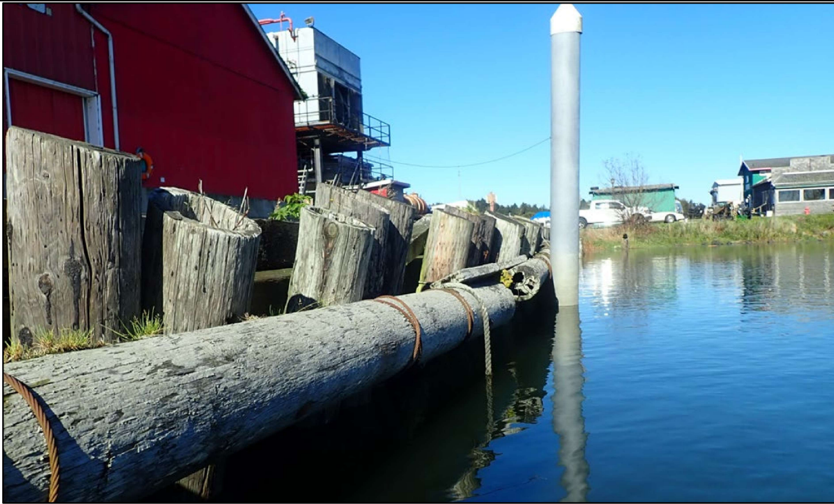
Figure 2. Damaged Bulkhead Wall
