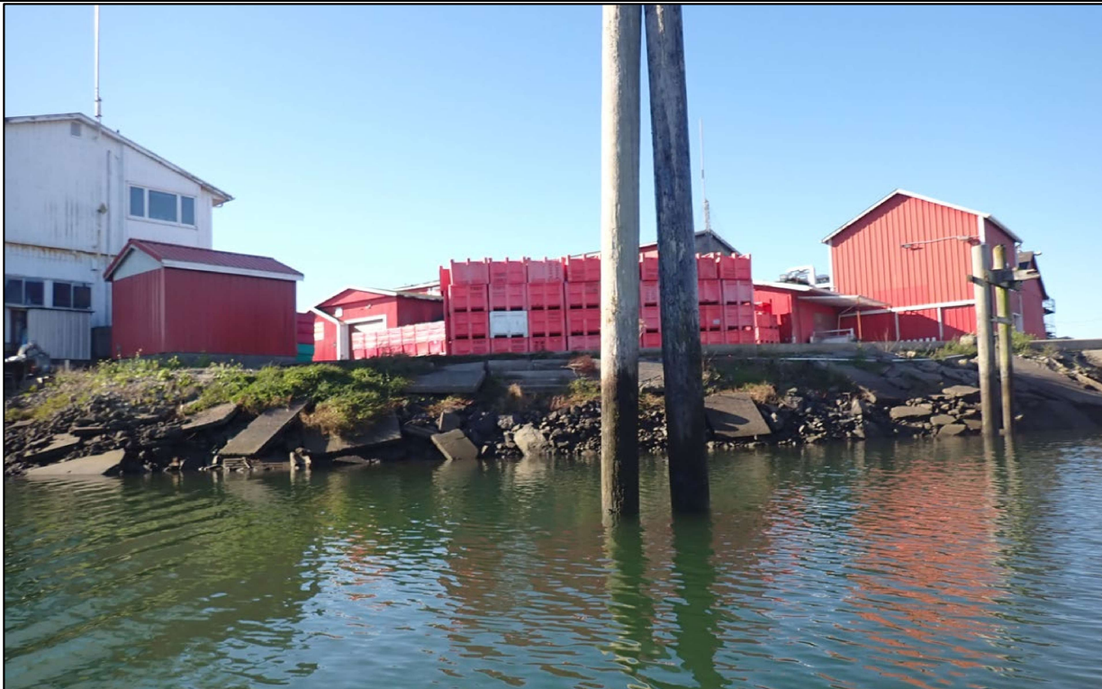
Figure 4. Riprap Shoreline to the South of the bulkhead Wall
