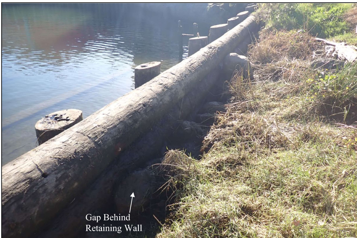
Figure 5. Retaining Wall to the North of the Bulkhead Wall
