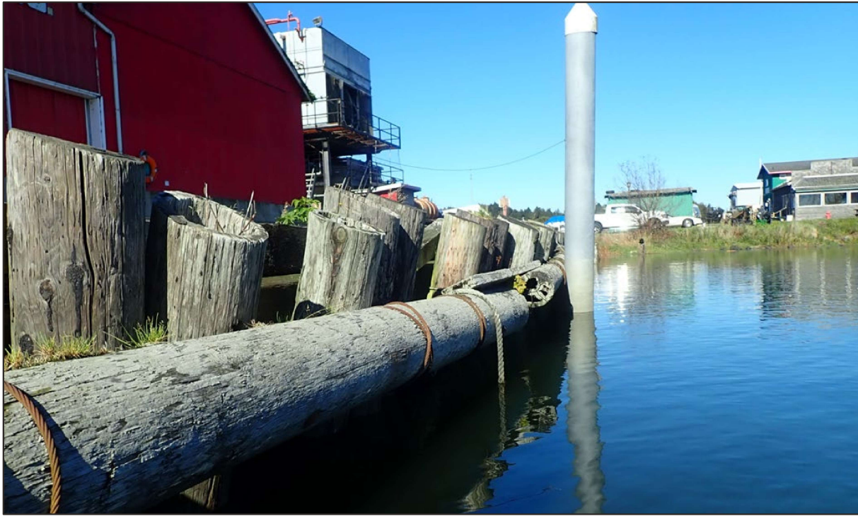
Figure 1. Damaged Bulkhead Wall
