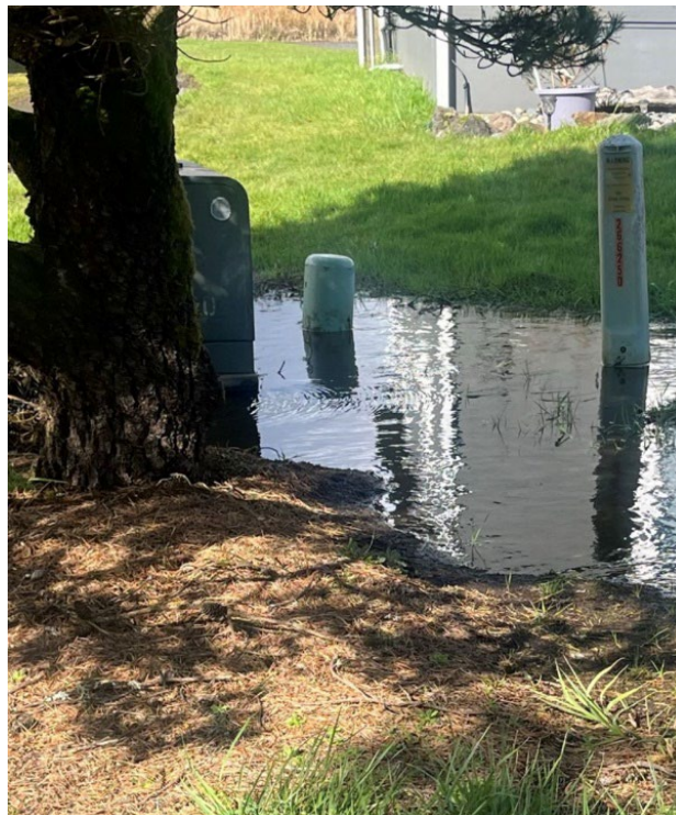
Photo 4. Inundated above ground infrastructure for electrical and telecommunication facilities in Pacific County, WA.
