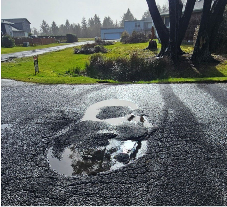
Photo 7. Collapsed culvert at Robert Gray Drive and Chattam Way
