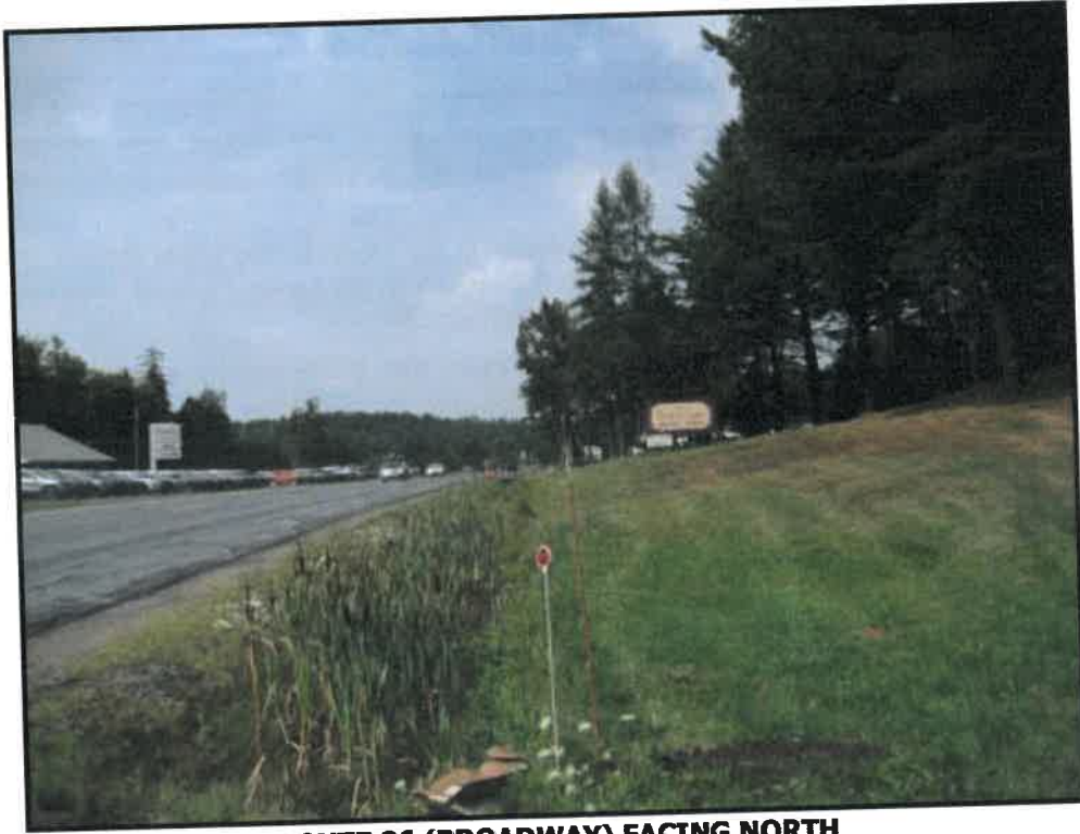
ROUTE 86 (BROADWAY) FACING NORTH
