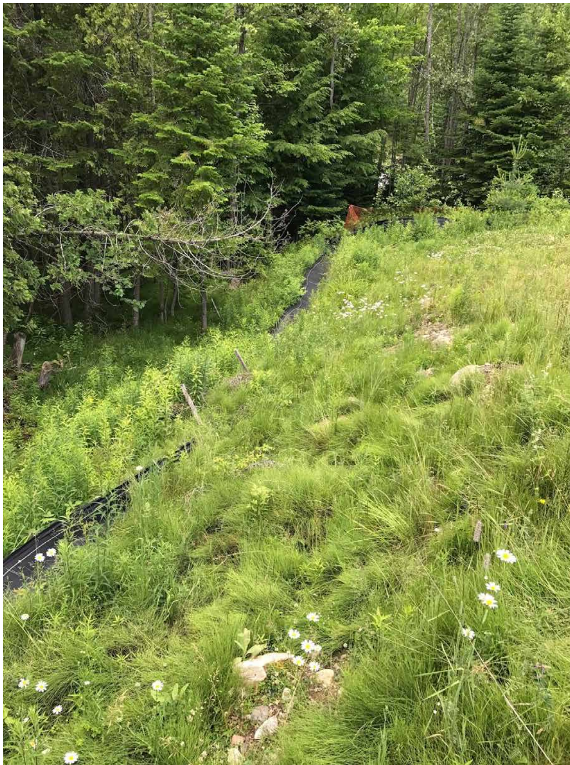
Photograph 2 Area of downed silt fence along south edge of property
