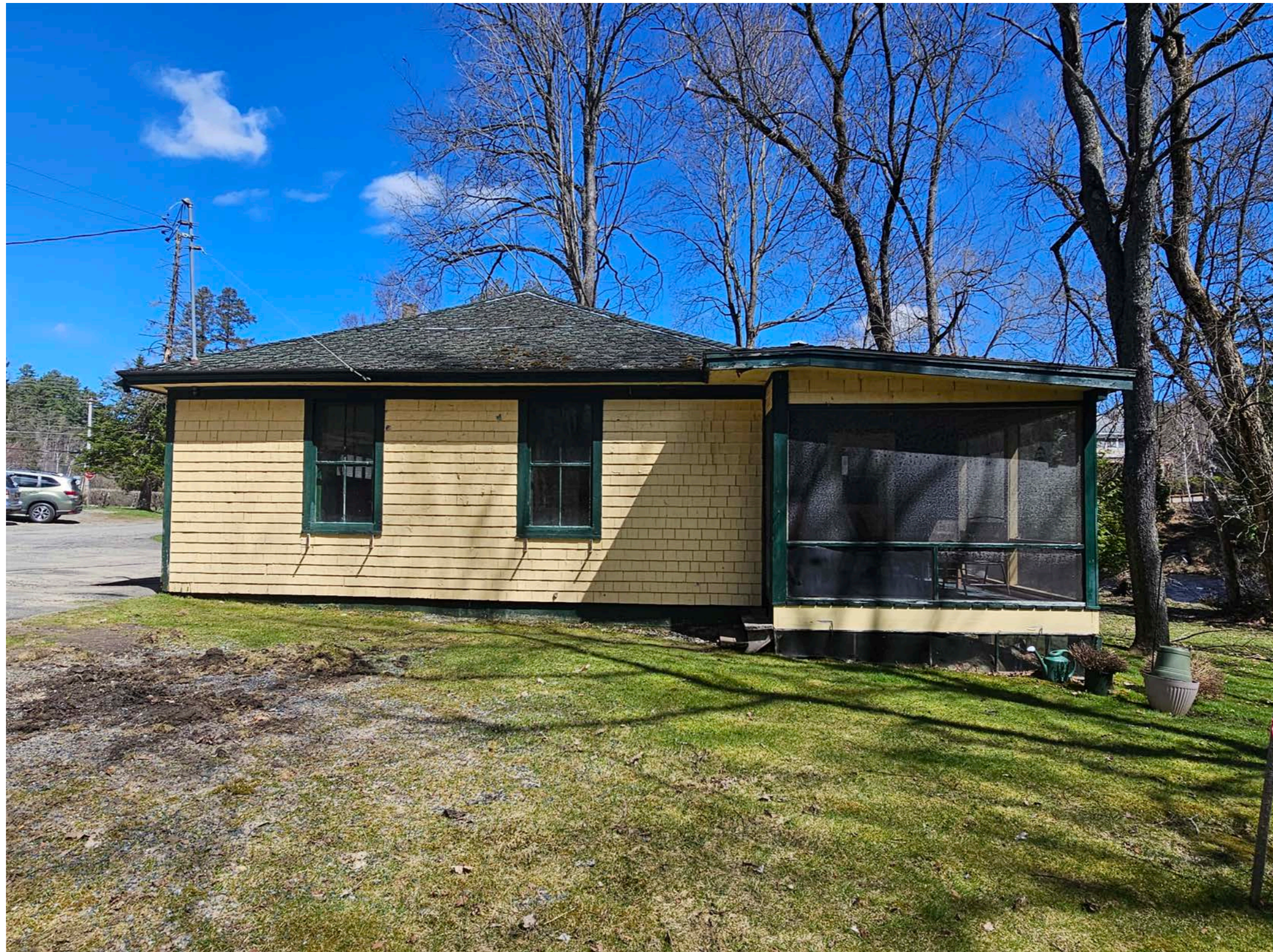
SIDE VIEW OF EXISTING TWO (2) BAY GARAGE TO BE REMOVED FOR NEW BUILDING 2 (LOCATED INSIDE TOWN OF ST. ARMAND, ESSEX COUNTY) TO CONSIST OF THREE (3) BAY GARAGE FOR TENANTS, WASTE PORTICO TO RIGHT SIDE OF GARAGE WITH PONY WALLS AT SIDES TO BLOCK VIEW OF BINS FROM STREET/RIVER & PORCH ON REAR OF BUILDING FOR TENANT USE. ONE (1) SINGLE UNIT APARTMENT ABOVE
