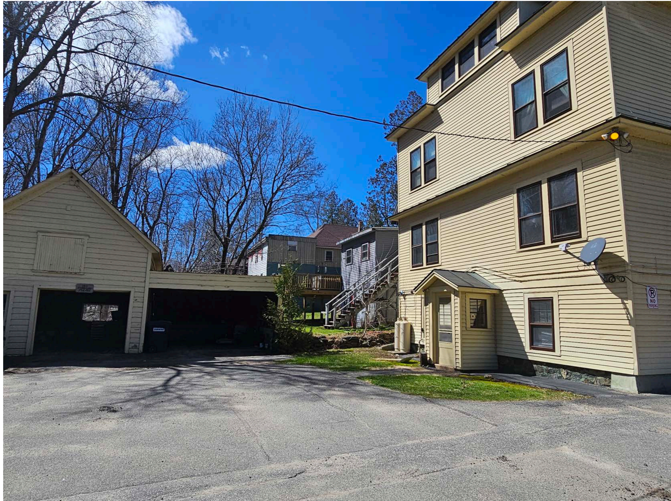
REAR VIEW OF EXISTING PRIMARY BUILDING (LOCATED IN TOWN OF ST. ARMAND / ESSEX COUNTY) EXISTING THREE (3) BAY GARAGE, SEEN PICTURED LEFT, TO BE REMOVED FOR NEW BUILDING 1
