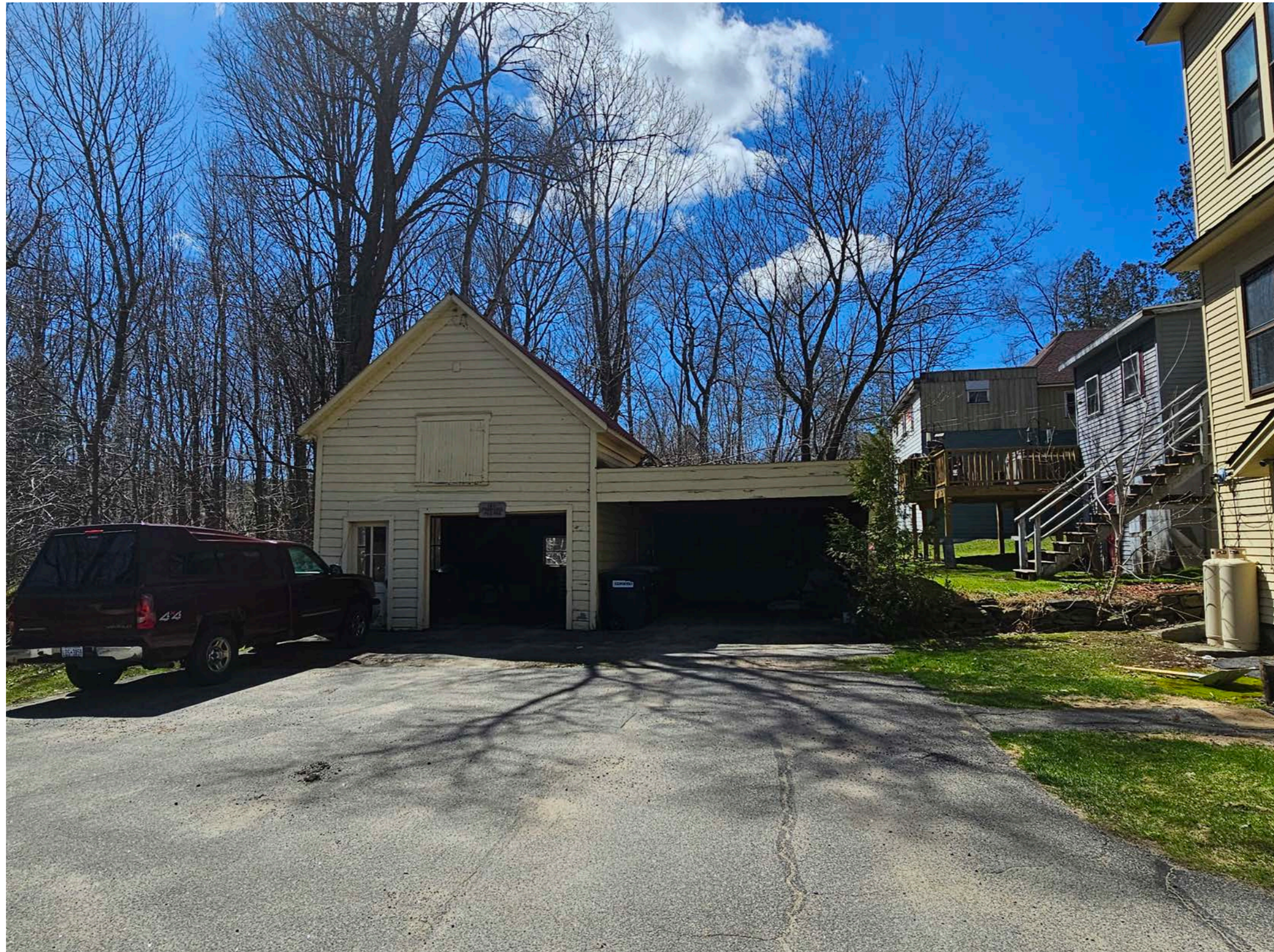
EXISTING THREE (3) BAY GARAGE TO BE REMOVED FOR NEW BUILDING 1 (LOCATED INSIDE VILLAGE LINE, FRANKLIN COUNTY) TO CONSIST OF THREE (3) BAY GARAGE FOR TENANTS, SINGLE UNIT APARTMENT IN REAR AND TWO (2) ADDITIONAL SINGLE UNIT APARTMENTS ABOVE
