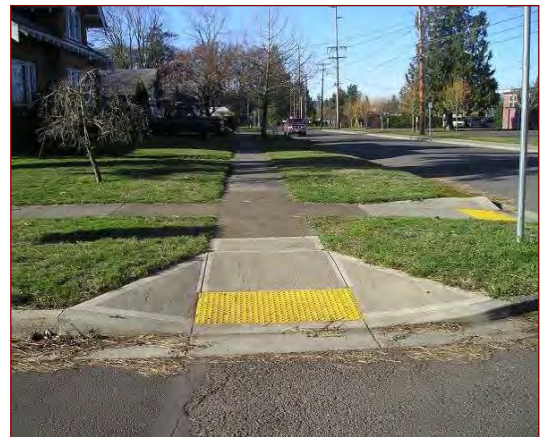
Example of an ADA-compliant curb ramp
