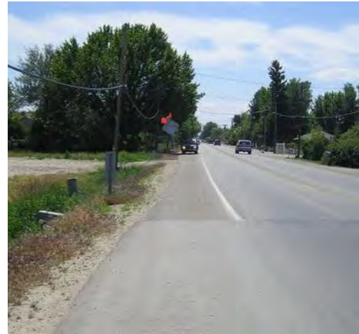
Shoulder bikeways are appropriate along wide rural roads where vehicles can avoid passing close to bicyclists
