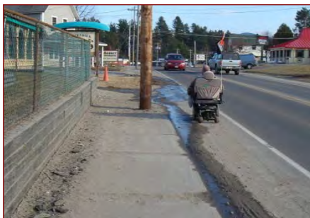
Figure 6. Narrow sidewalks are often blocked by utilities and do not provide adequate pedestrian space
