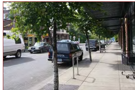
Figure 7. A well-designed sidewalk provides plenty of pedestrian space, as well as trees, bike parking, and a planter zone
