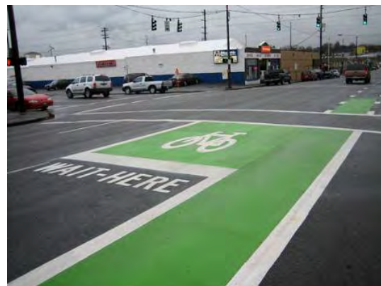
Bike boxes have been installed at several intersections in Portland, OR where right-turning motorists conflict with through bicyclists
