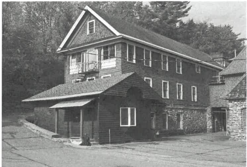
Cold Storage Building
