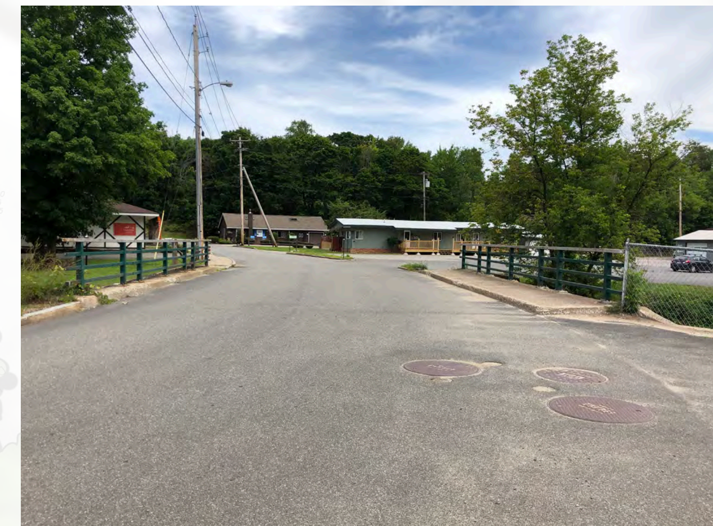
WOODRUFF STREET BRIDGE
