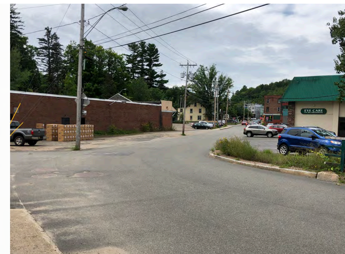
WOODRUFF STREET (BRIDGE - WEST)
