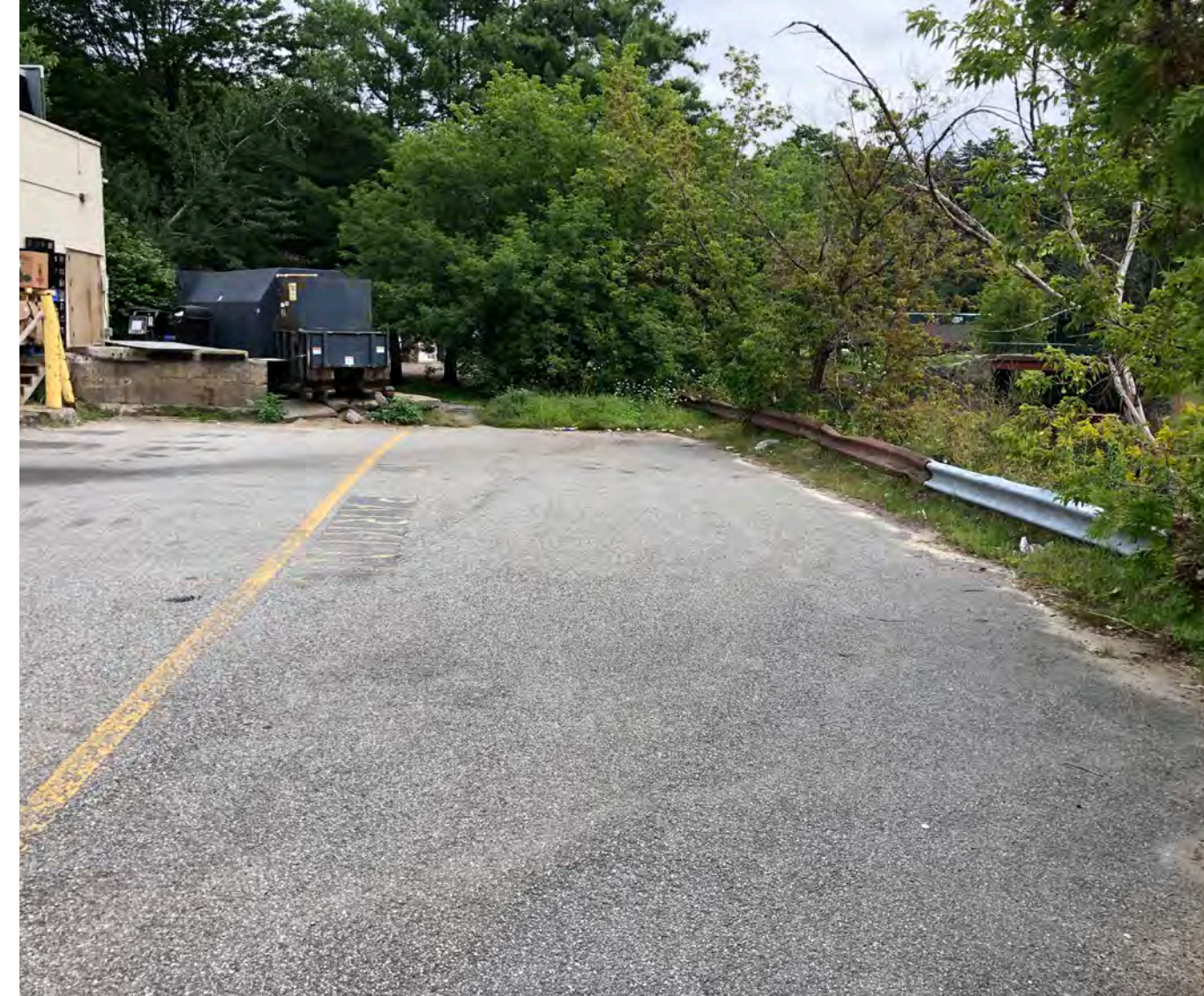
Existing Guard Rail at Tops
