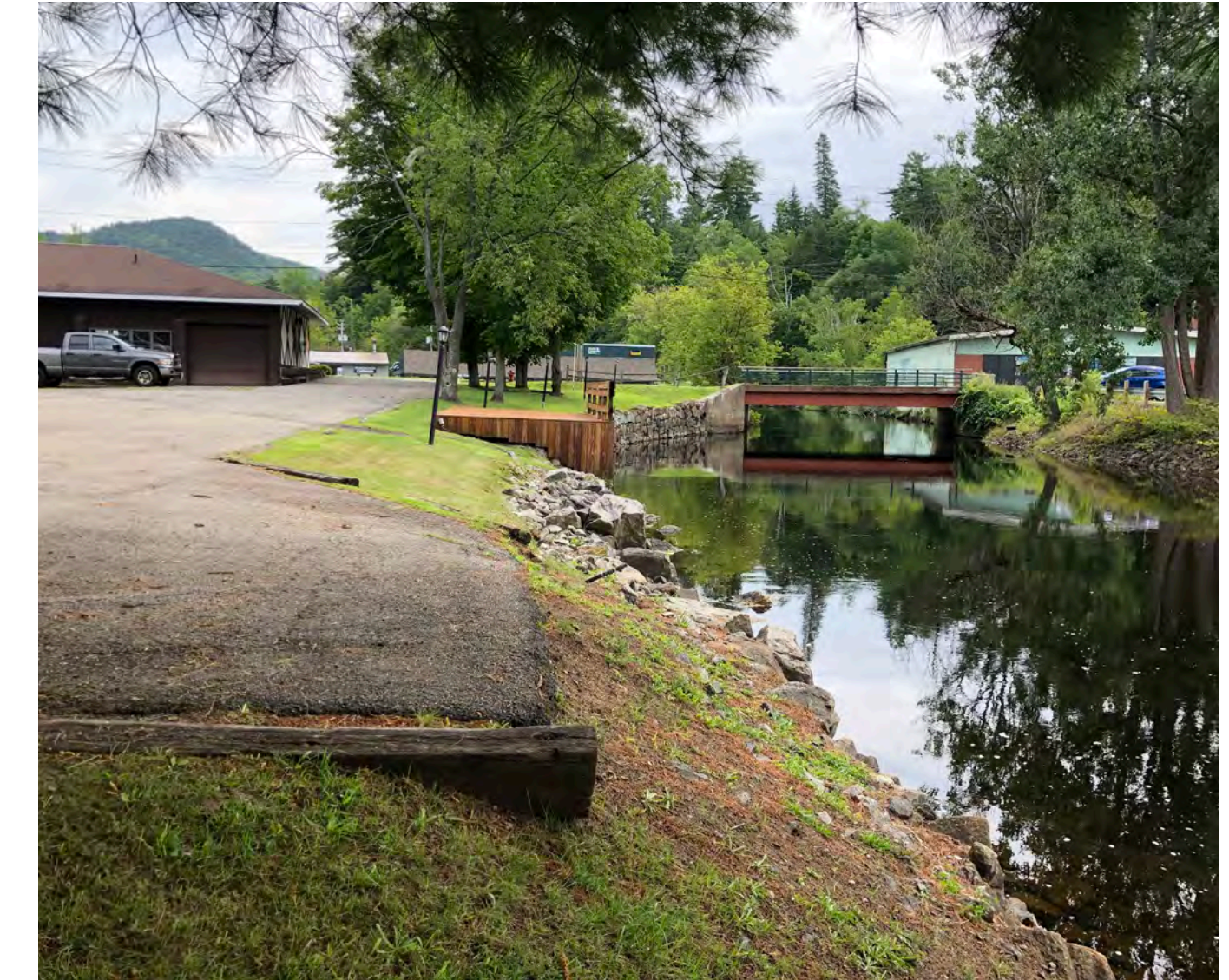
Existing Slope Conditions
