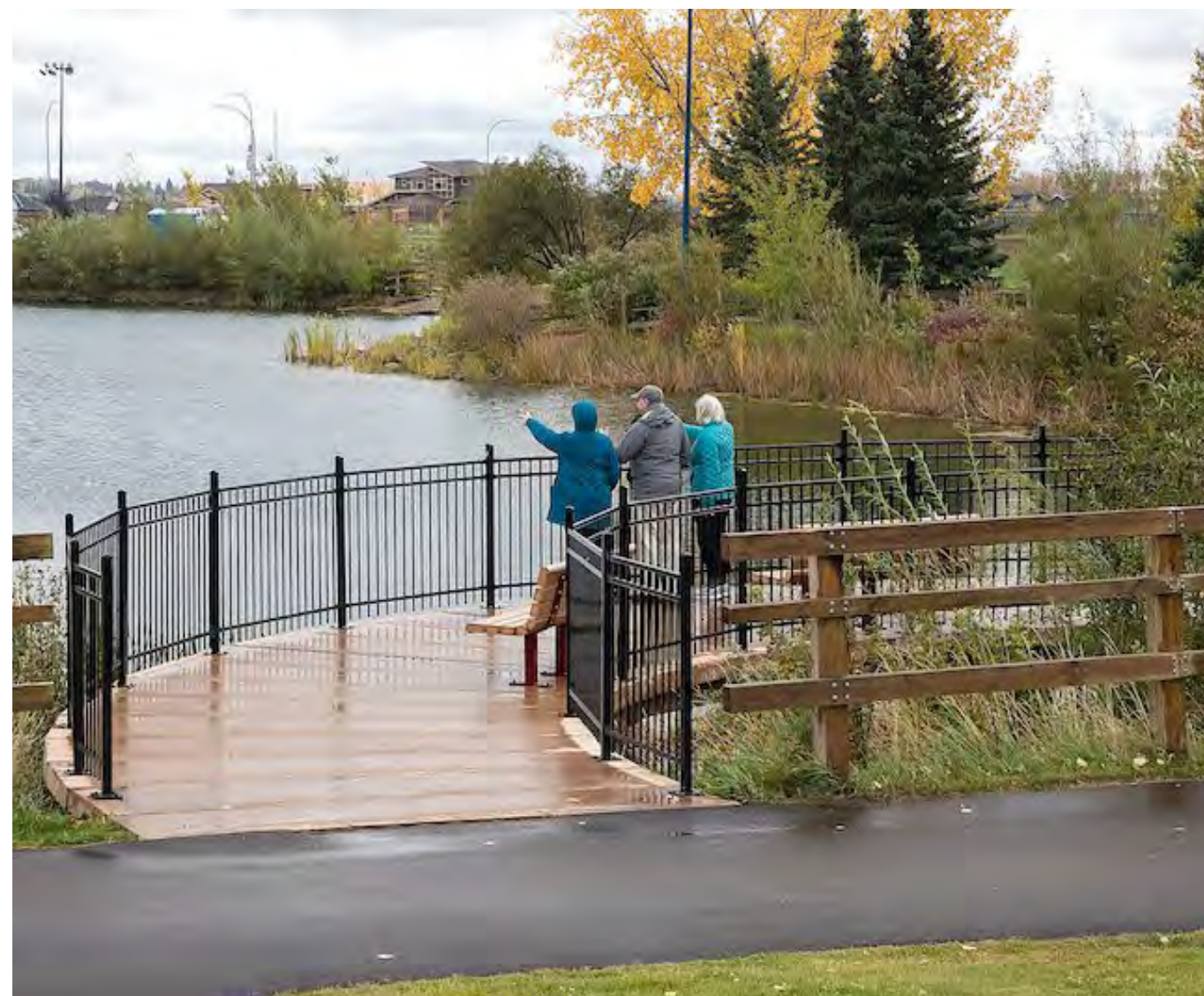
PermaTrak Boardwalk (concrete)
