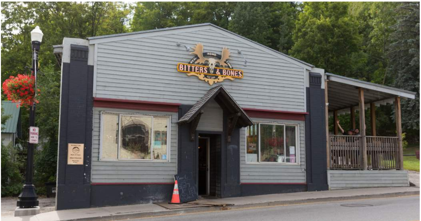
Existing Conditions – Front View from Broadway
