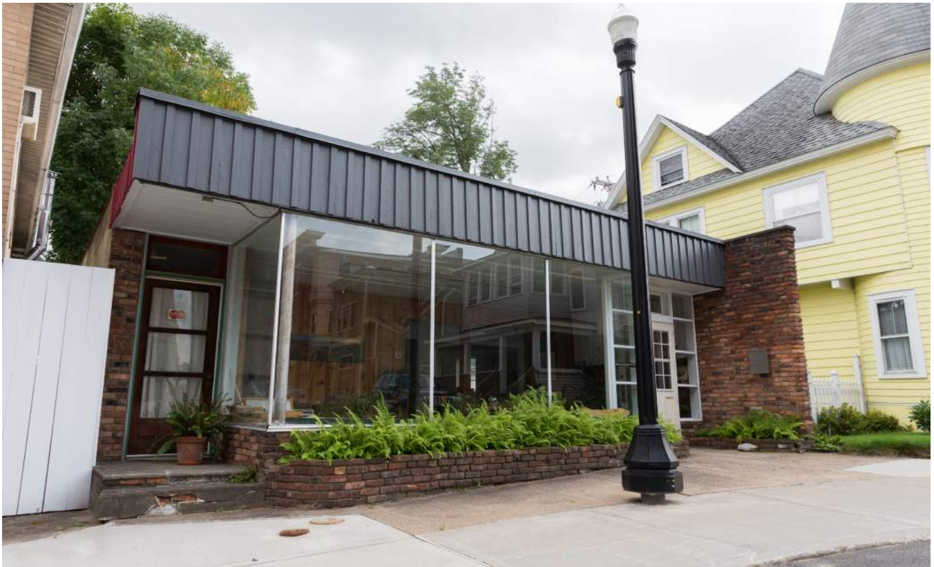
Existing Conditions – Front View from Academy Street
