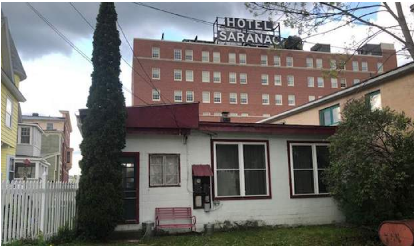
Existing Conditions – Rear View
