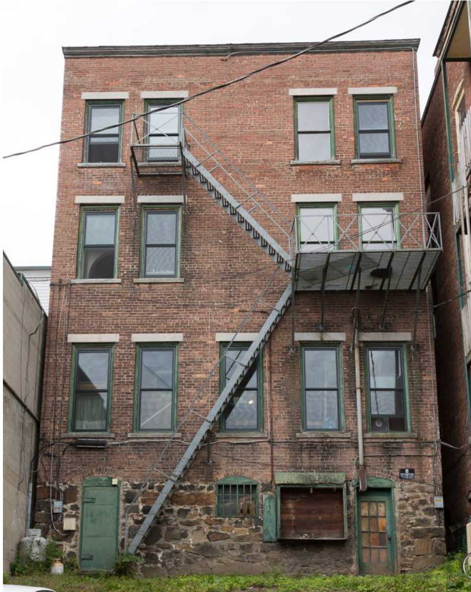
Existing Conditions – Rear View from Dorsey Street Lot
