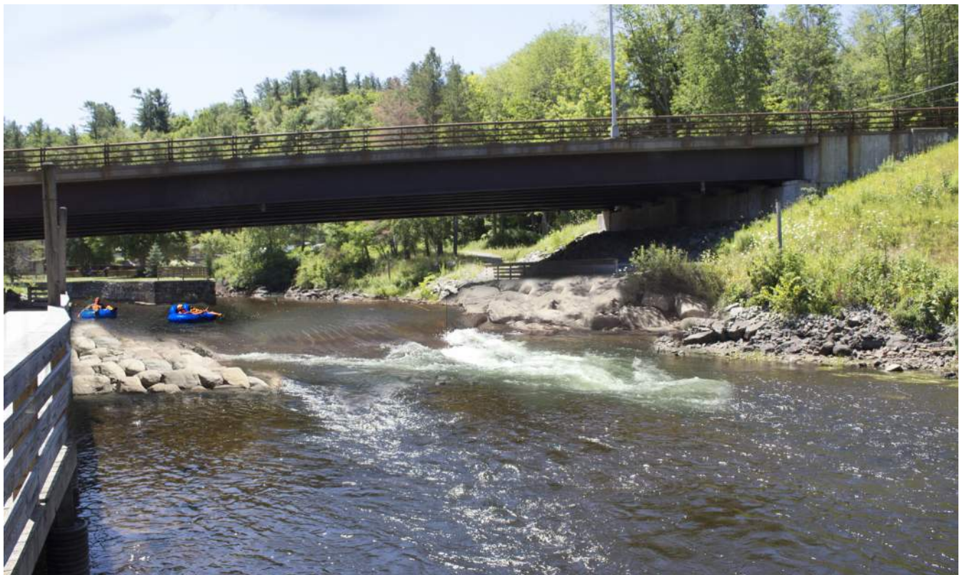
Saranac Lake Whitewater Park-Proposed Condition. Rendering of Kayakers Looking South Along Saranac River
