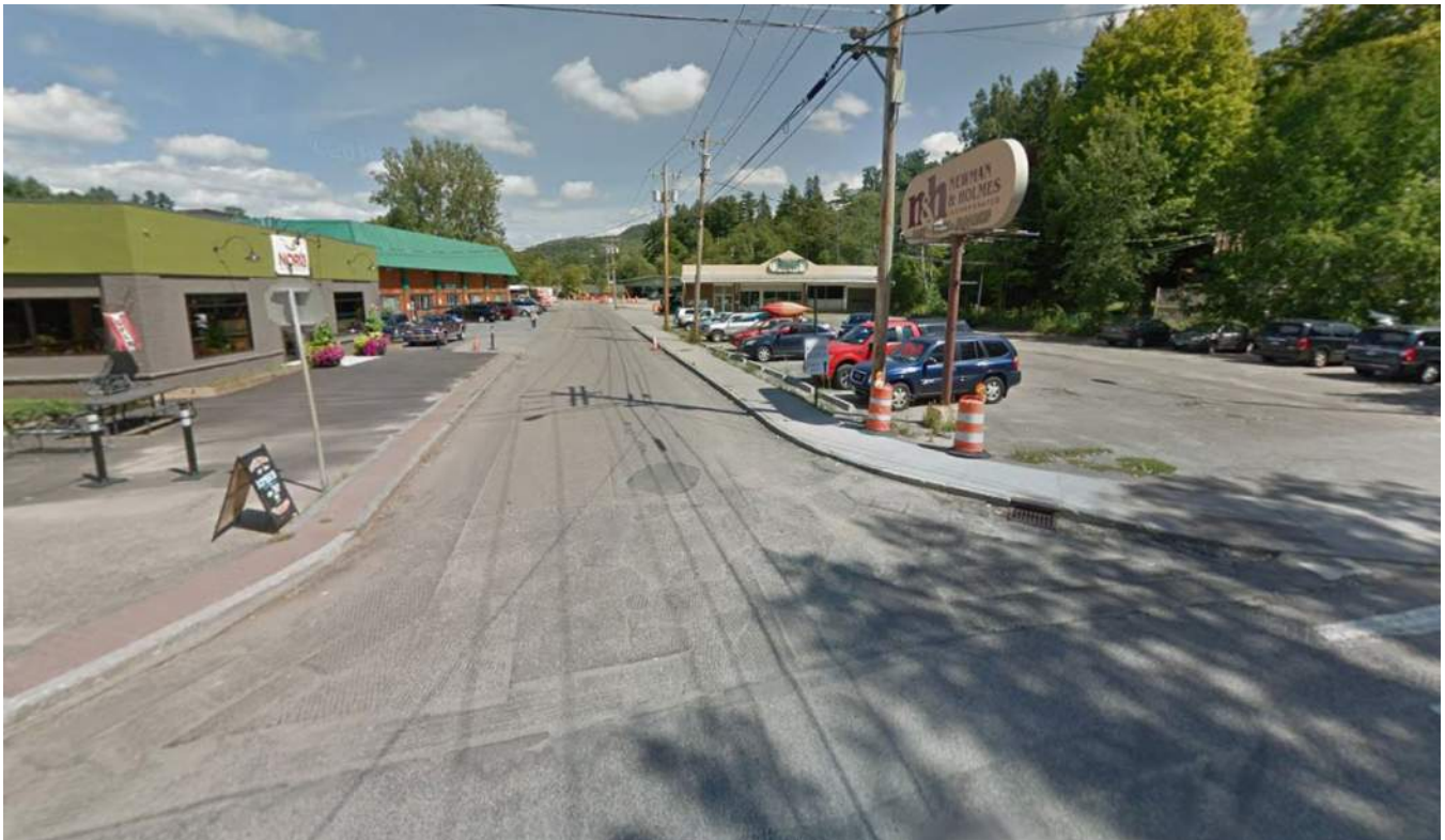
Woodruff Street East-Existing Condition
