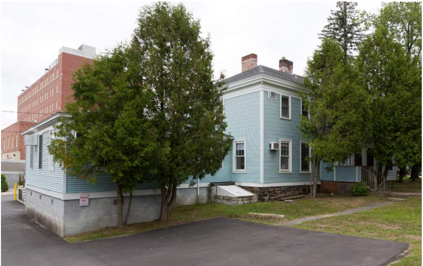
Existing Conditions – Rear View Trudeau Building
