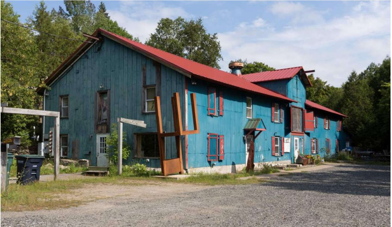
Existing Conditions - Front view from Cedar Street
