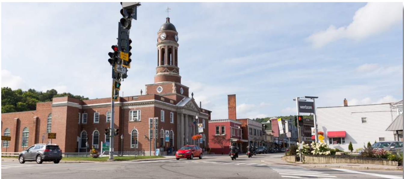
Town Hall at the intersection of River Street and Main Street
