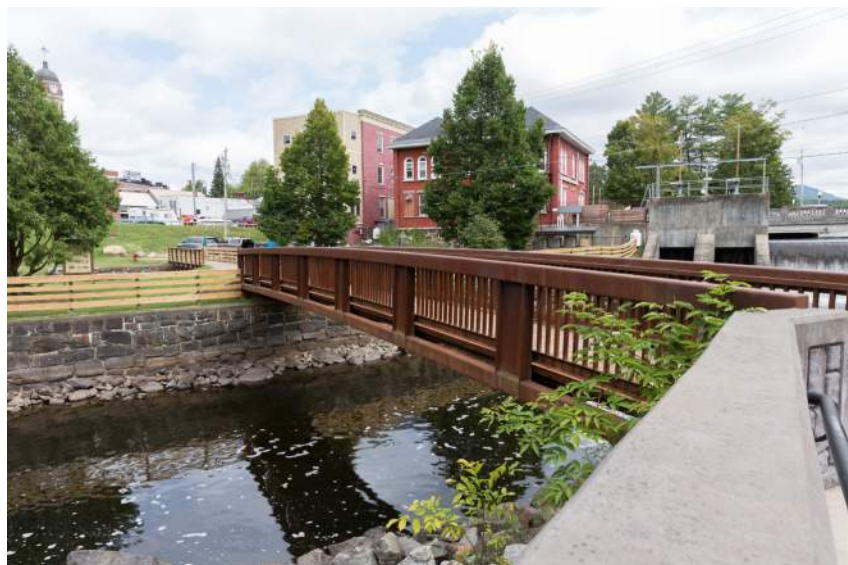
Pedestrian bridge at Hydro Point Park
