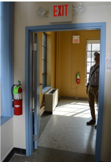
2 nd floor – Modern door to Stairhall
