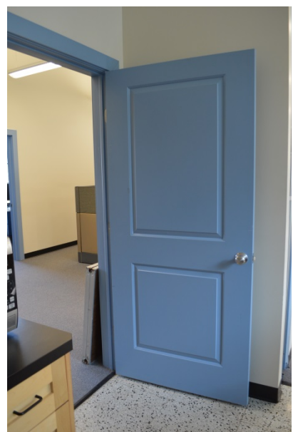
3 rd floor - View of typical modern door.
