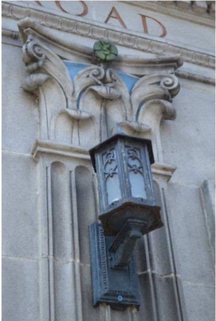
Original cast iron light fixture.
