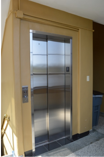
View of infilled elevator opening
