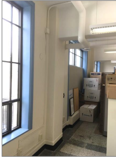
First floor–Exterior plaster walls Note surface applied conduit.
