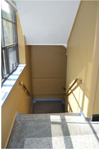
Stair run to mid-rise landing.
