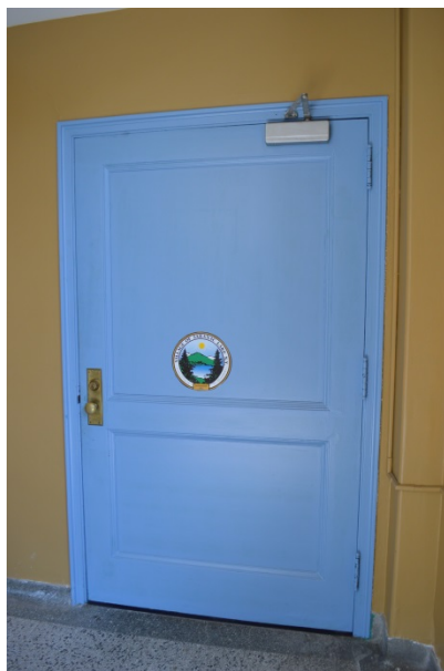
3 rd floor - Original metal clad door.
