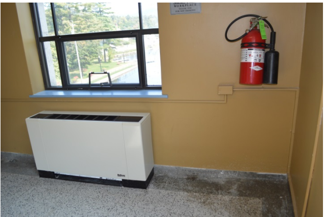
2 nd floor – View of east wall showing alterations
