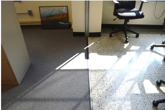
3 rd floor - Area of floor showing terrazzo & carpeting
