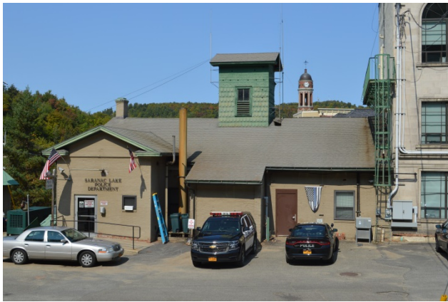
Front (south) façade of Police Dept-note proximity of cars
