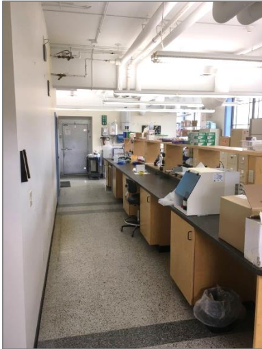
First floor–Terrazzo flooring with Borders interrupted by new partitions.
