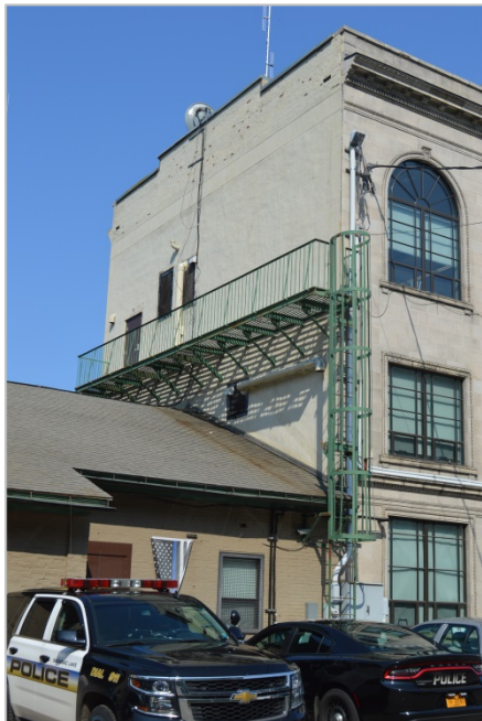
View show infilled windows on West wall.
