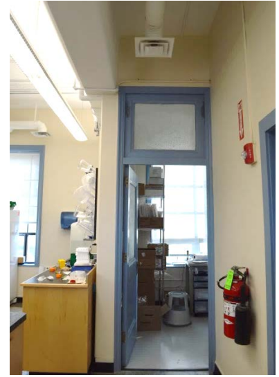
2 nd floor –Original door & transom
