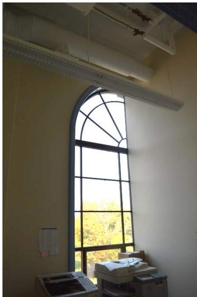
3 rd floor - View of bisected window
