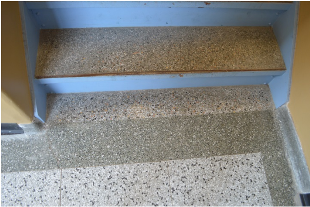
2 nd floor –View of three terrazzo colors & stair structure
