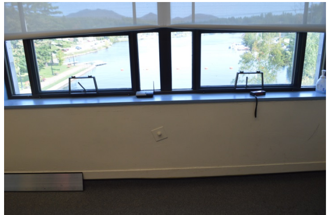
3 rd floor - Detail view of modern replacement window.
