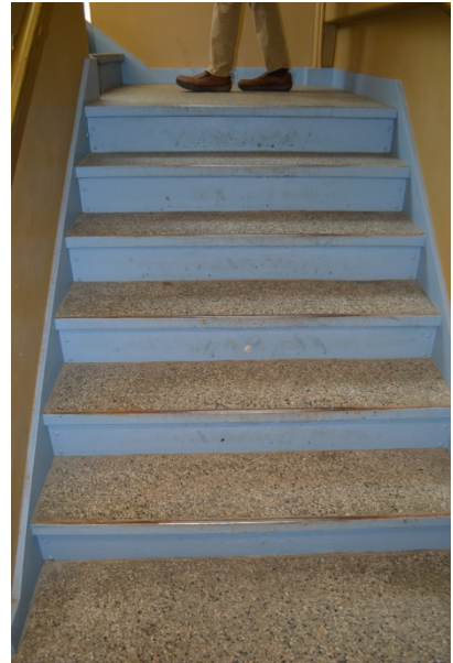
View of typical prefab stair.
