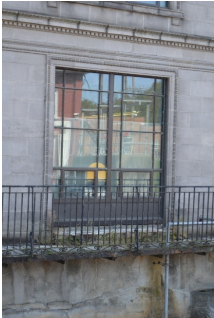
Original wrought iron balcony along north elevation
