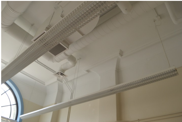
3 rd floor - Original flared pier capitals & plaster cornice.
