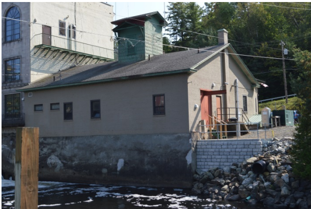
View of north side showing current fenestration pattern.
