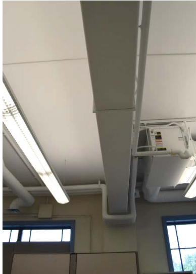
2 nd floor – North wall showing beams obscured by pipes & mechanical equip.
