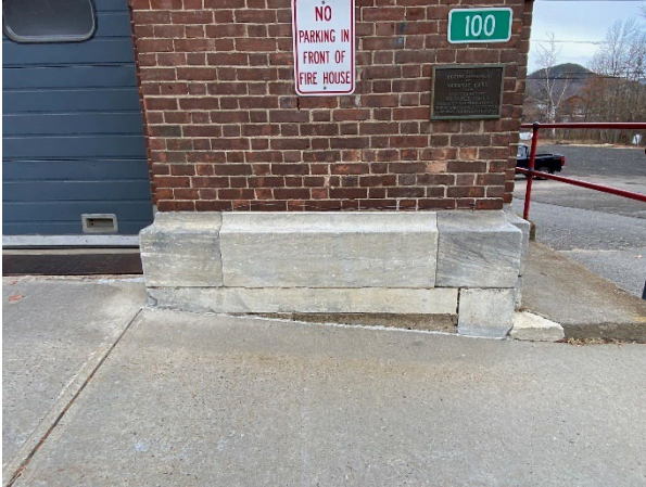
Cut & dressed marble foundation.
