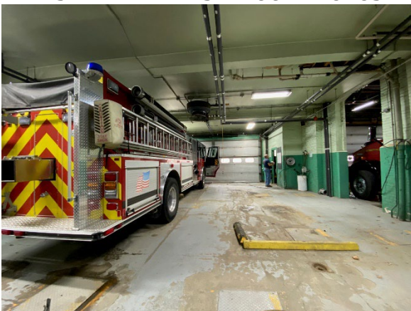
1 st floor garage looking towards front (west) wall.
