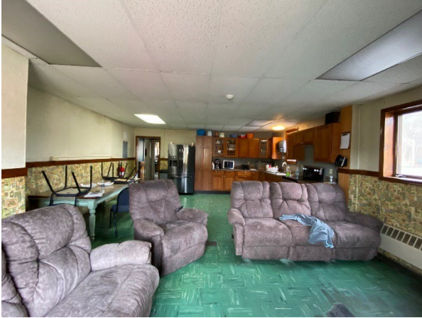
2 nd floor Kitchen/Lounge space with mid 20 th c. wall, ceiling and floor finishes. Cabinetry is 21 st century and in good condition.
