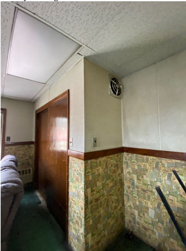
Closet built into SE corner of Kitchen is modern with hollow core sliding doors. Masonite paneling covered with wallpaper.
