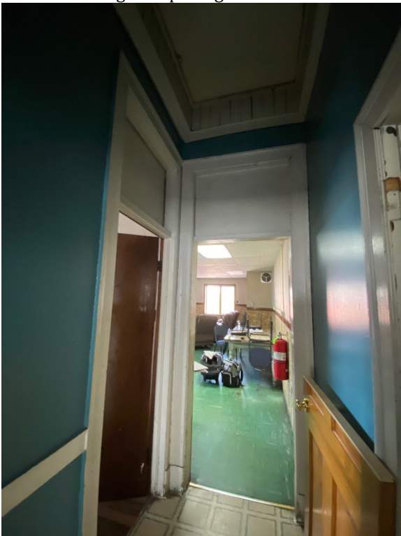
Central 2 nd floor short hallway retains original trim elements at doorways.
