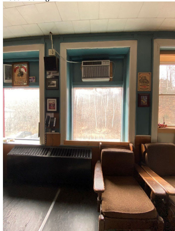
View of centered windows on front wall of Day Room with plywood infills and fixed window units replacing orig. double hung sash.
