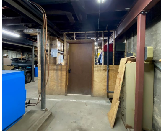
View of north wall of former coal bin, now used for secured gear storage.
