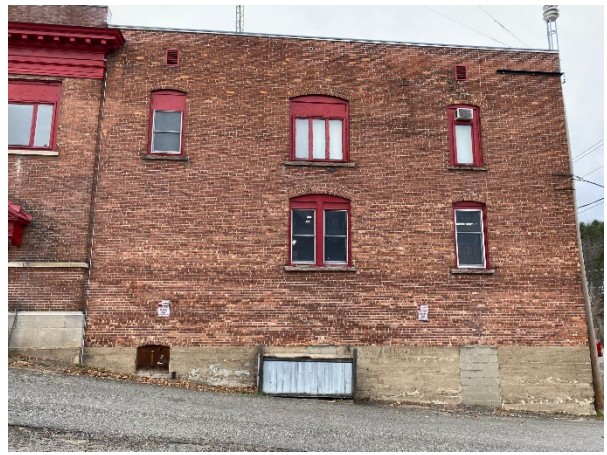
South elevation with altered window openings.
