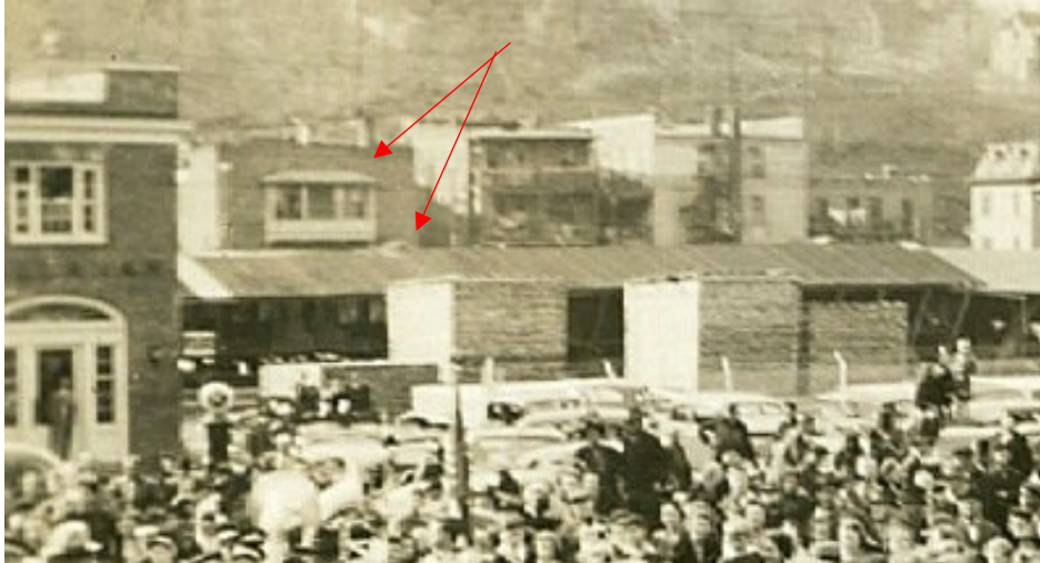
View looking west from Depot Street, with rear elevations of Broadway bldgs. Note 2 nd story bay window & gable ridge of NE addition.
