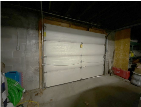
Modern overhead garage door on rear (east) wall.
