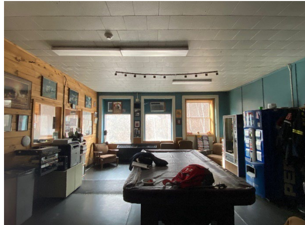
View to west (front) wall in Day Room where orig. windows and doors to former balcony have been infilled & replaced.
