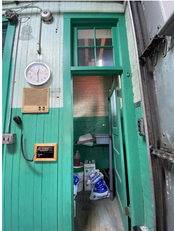
Front SW closet with original beaded board partition, paneled door & transom window.
