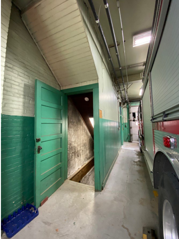
Stair case along south wall with orig. beaded board finishes & paneled door.
