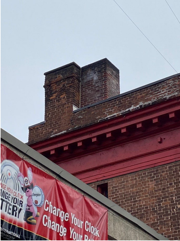
Metal entablature returned on north elevation. Note brick parapet & orig. chimney with new boiler chimney added next to it.
