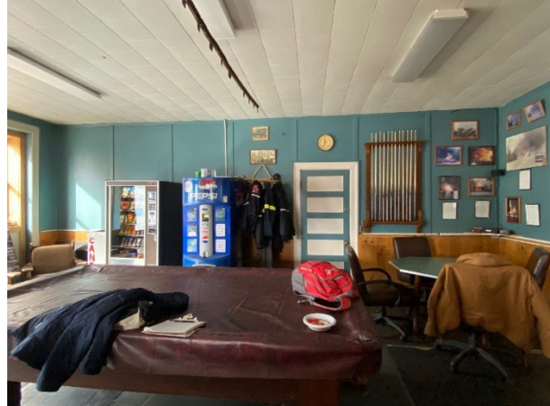
North wall of 2 nd floor Day Room showing paneled wall sheets with battens & original 5-paneled door to closet.
