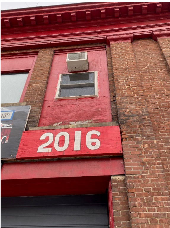
Second floor door & window openings infilled with painted plywood, replacement units & a/c
