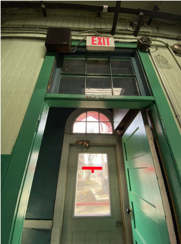
View of side entry vestibule with original paneled door & transom windows.
