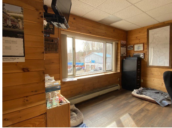
Large original window opening infilled & framed down with smaller plate glass and casement windows.
