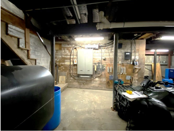
Shiplap board partition wall at bottom of stairs in SW corner – former coal bin. Note new elect. panel.
