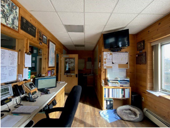
Subdivided Dispatch Room finished all in knotty pine horiz. boards with acoustical tiled ceiling.
