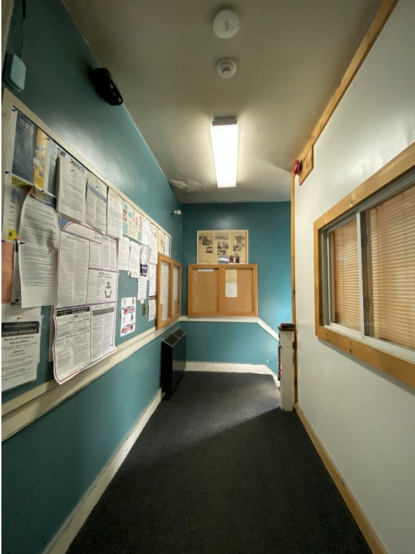
Stair hall has wall-to-wall commercial carpeting but orig. wood baseboard intact on 3 of 4 walls.
