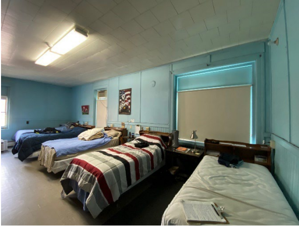
South and east walls of Bunk Room show how original window openings have been retained but have modern replacement units.
