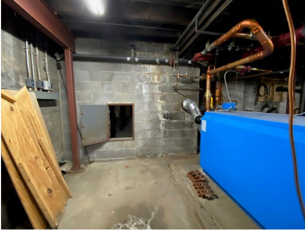
View of wall of hose tower with access door. Note new boiler exhausts into new chimney built within hose tower.
