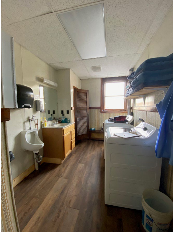
Bathroom/shower/laundry facilities on 2 nd floor positioned along north wall. Window is framed down from original openings size.
