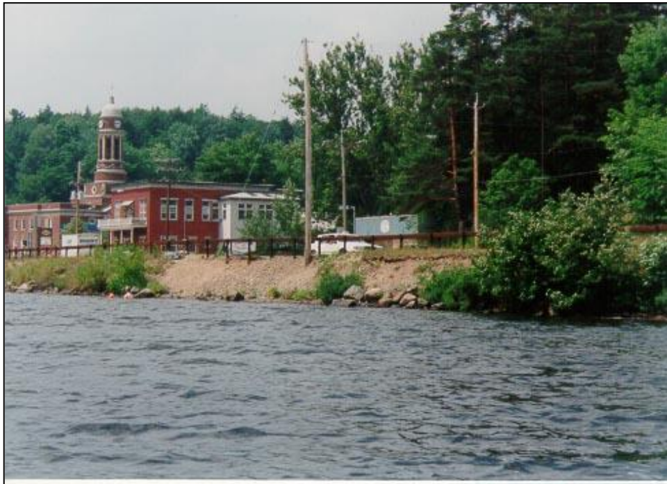
Erosion along River Street
