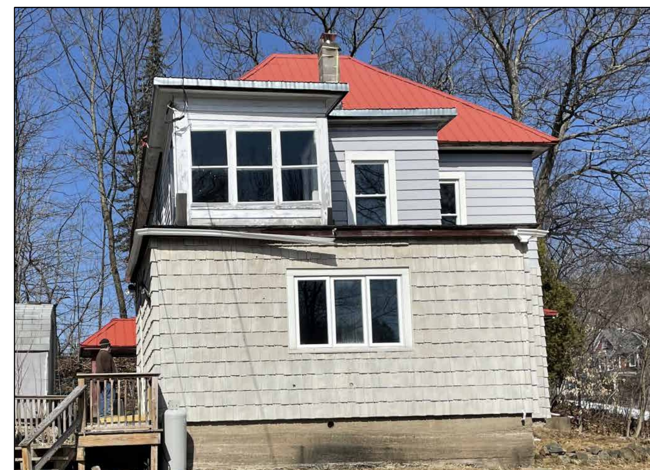
2 SIDE OF HOUSE - FACING MC CLELLAND ST. - EXISTING CONDITIONS SCALE: 3/16" = 1'-0"
