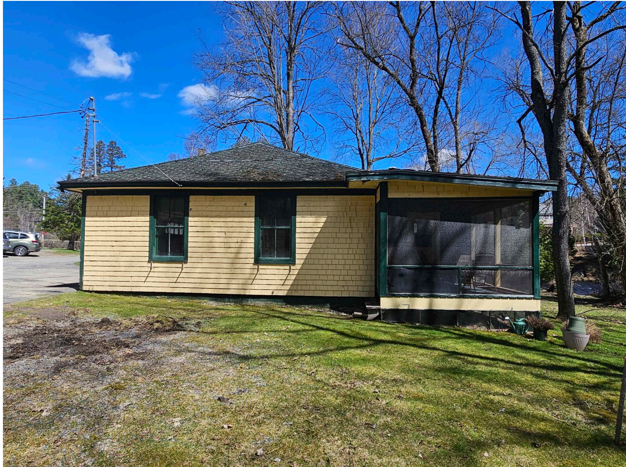
SIDE VIEW OF EXISTING TWO (2) BAY GARAGE TO BE REMOVED FOR NEW BUILDING 2 (LOCATED INSIDE TOWN OF ST. ARMAND, ESSEX COUNTY) TO CONSIST OF THREE (3) BAY GARAGE FOR TENANTS, WASTE PORTICO TO RIGHT SIDE OF GARAGE WITH PONY WALLS AT SIDES TO BLOCK VIEW OF BINS FROM STREET/RIVER & PORCH ON REAR OF BUILDING FOR TENANT USE. ONE (1) SINGLE UNIT APARTMENT ABOVE
