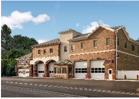
Purchase Fire Station; Purchase, NY Renovations & Addition 2021 Notable Design Award, Firehouse Magazine
