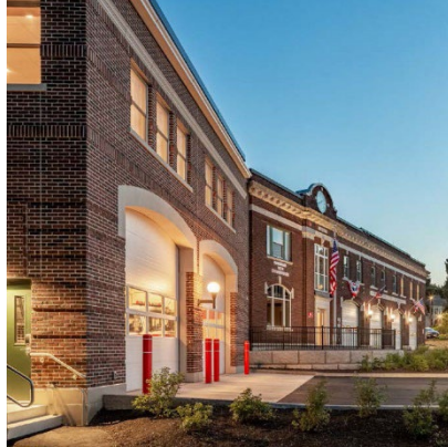
Hartford Fire Station Augusta, ME (1) Renovations & Additions 2019 Silver Award, Firehouse Magazine & A 2019 Honor Award from Maine Preservation
