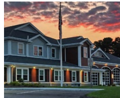
Carver Public Safety Facility; Carver, MA (3) New Construction 2017 Gold Award, Firehouse Magazine
