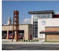
City of Yonkers Fire Station 1. Yonkers, NY (4) New Construction 2020 Notable Design Award, Firehouse Magazine
