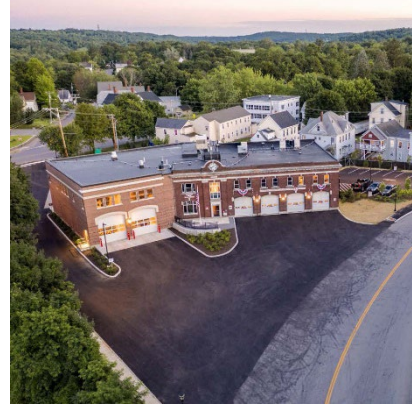
Hartford Fire Station Augusta, ME (1) Renovations & Additions 2019 Gold Award, F.I.E.R.O. Fire Station Design Symposium
