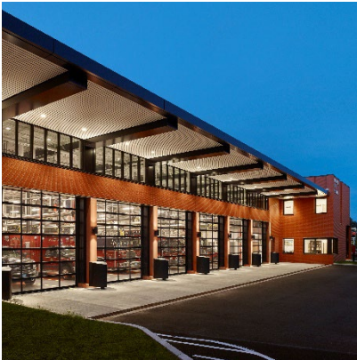
Walpole Central Fire Station, Walpole, MA (2) New Construction, Consolidation 2019 Gold Award, F.I.E.R.O. Fire Station Design Symposium
