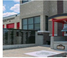
South River Fire Headquarters; South River, NJ New Construction 2018 Notable Design Award, Firehouse Magazine
