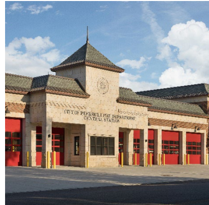
Peekskill Fire Headquarters, Peekskill, NY New Construction, Consolidation 2019 Bronze Award, F.I.E.R.O. Fire Station Design Symposium
